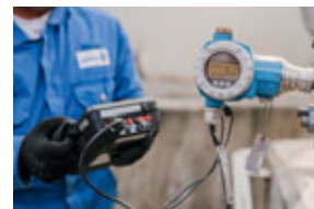
Safety checks at Pasir Gudang
