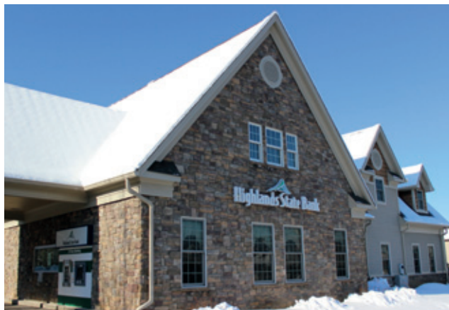
Highlands State Bank Headquarters, Vernon NJ
