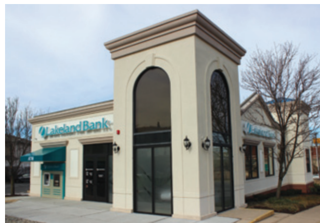
Clifton Branch Office
