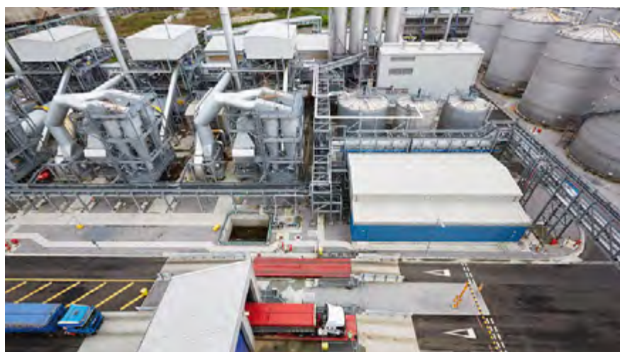
Vivergo’s bioethanol plant in Hull, the reopening of which was announced in February 2021.
