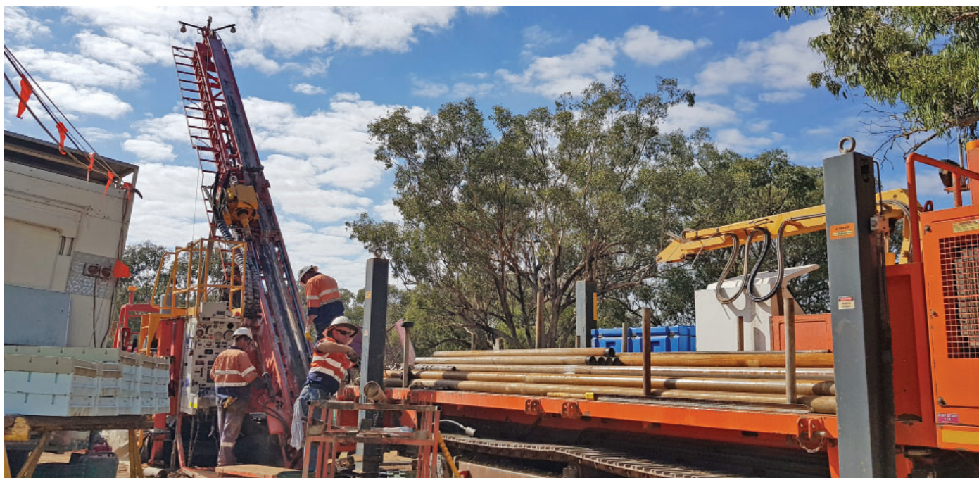
Figure 3 – Pine Ridge drilling April 2019
