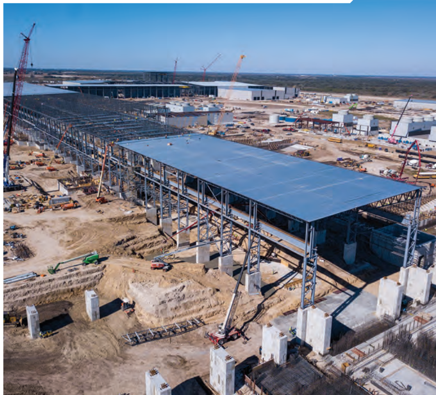
Sinton Steel Mill Construction
