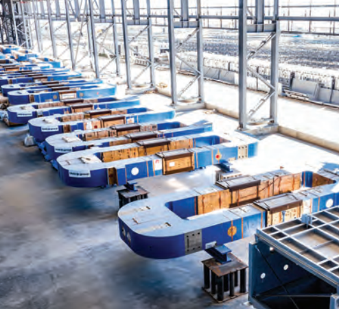
Sinton Steel Mill, Mill Stands Staged for Installation
