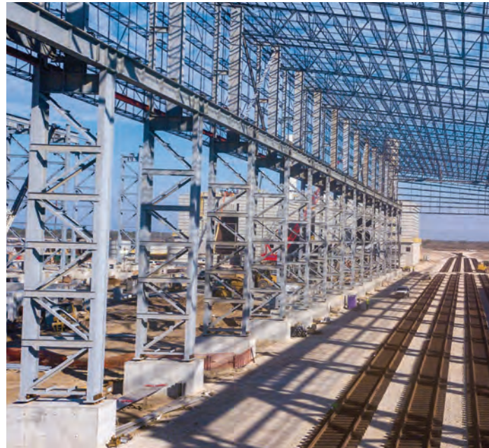
New Sinton Steel Mill Future Scrap Bay
