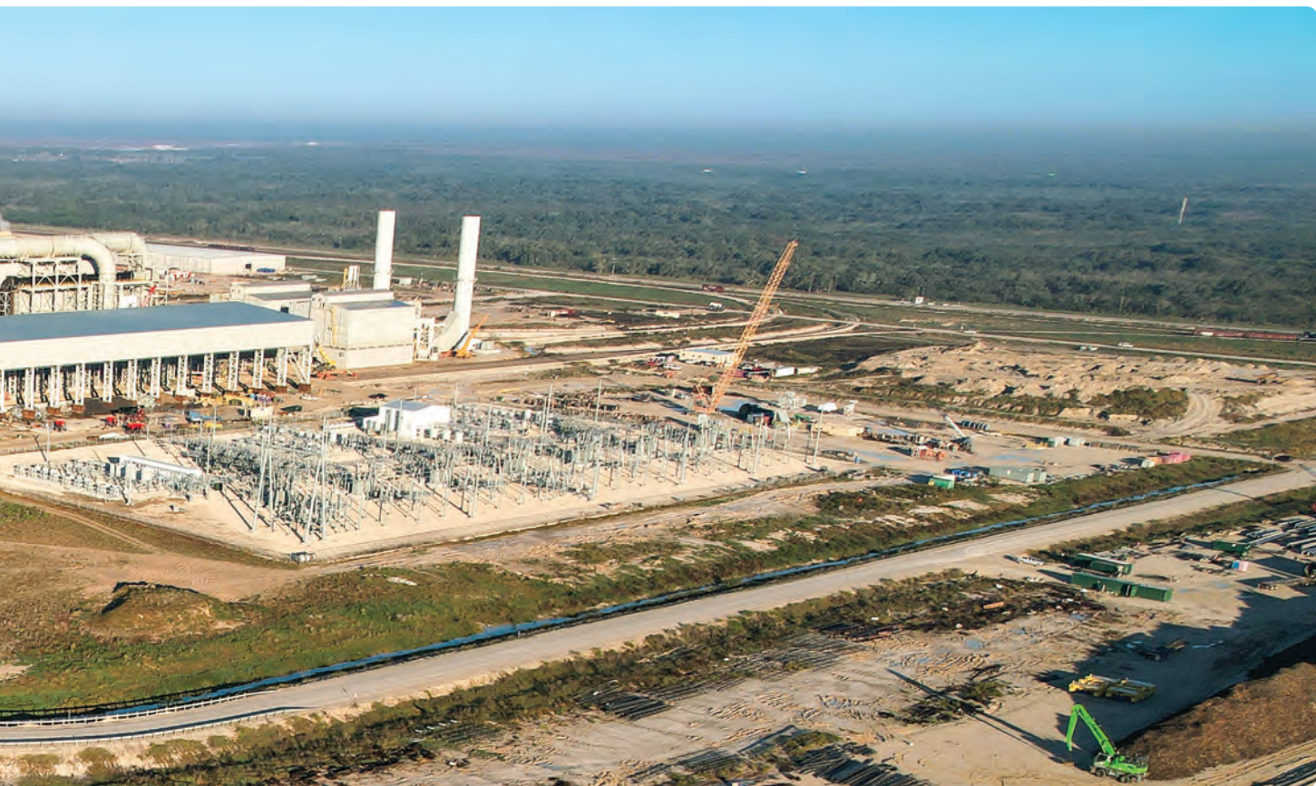
Sinton Steel Mill | December 2021
