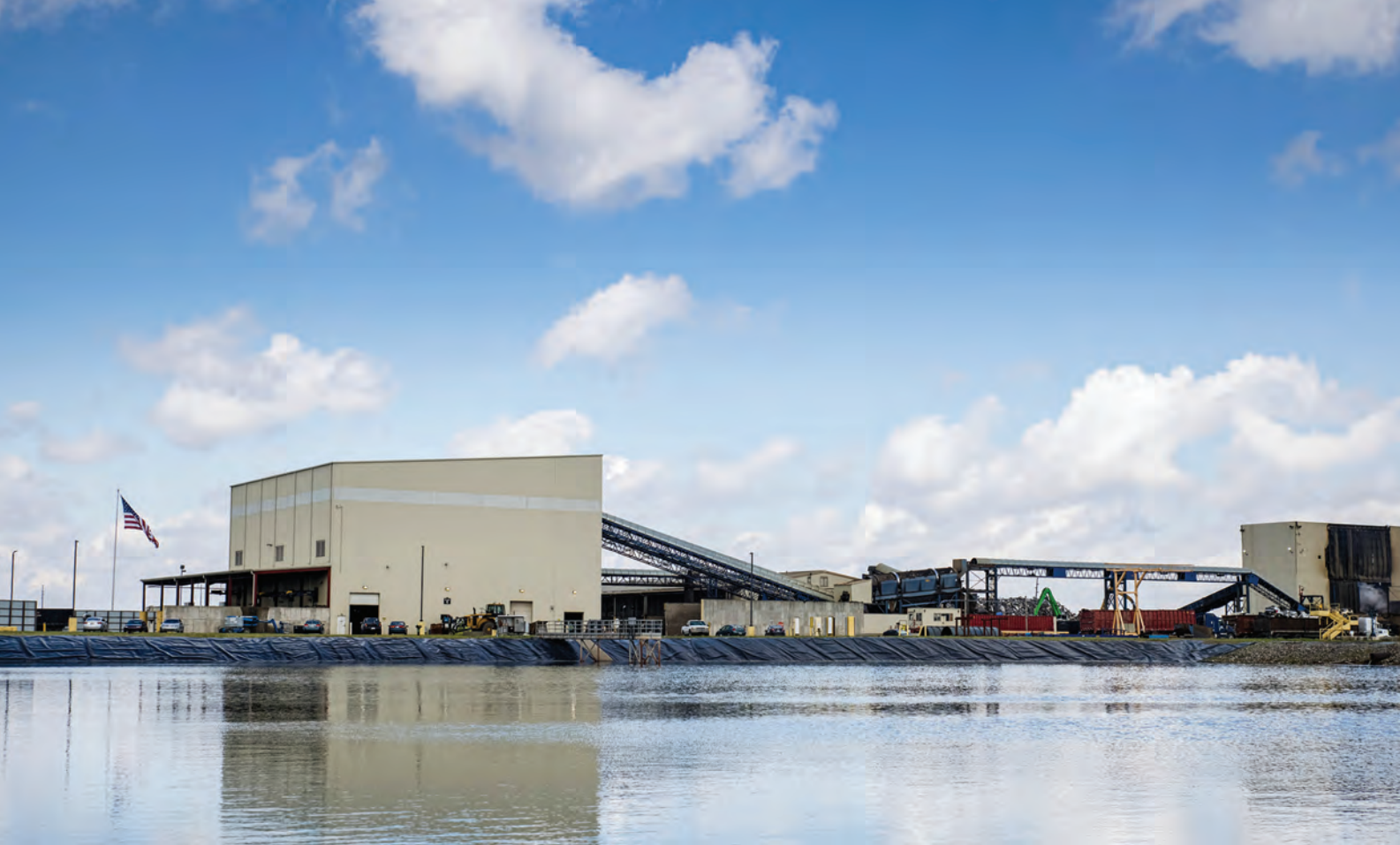
OmniSource Recycling Facility
