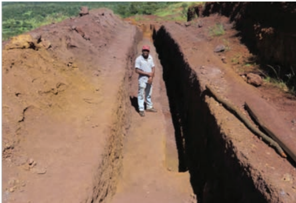
One of several excavated trenches for 66 tonne bulk sample collection, March 2015.
