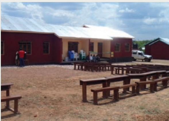
Preparations for the handover of the second pair of teachers houses constructed by Peak for the Ngwala Primary School, November 2014.
