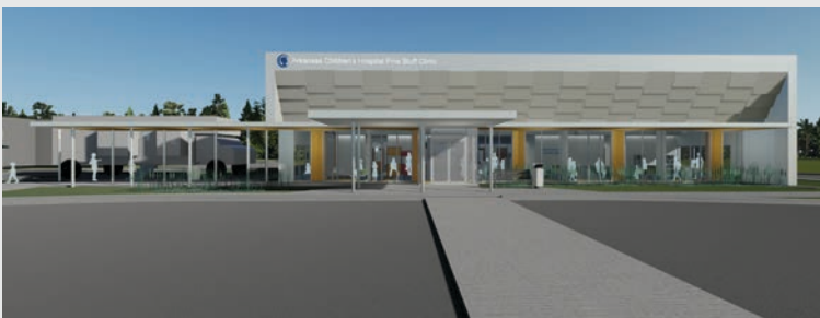
Arkansas Children's Hospital Pine Bluff Clinic
