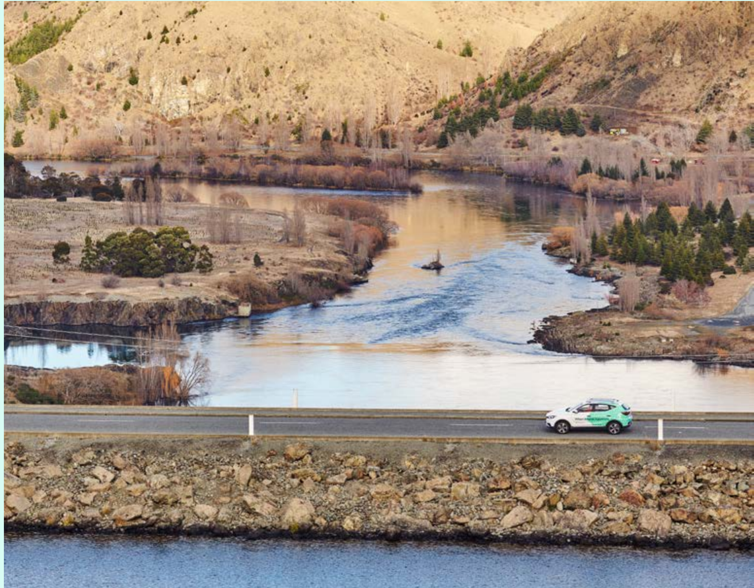
Benmore Hydro Power Station, Otematata.
