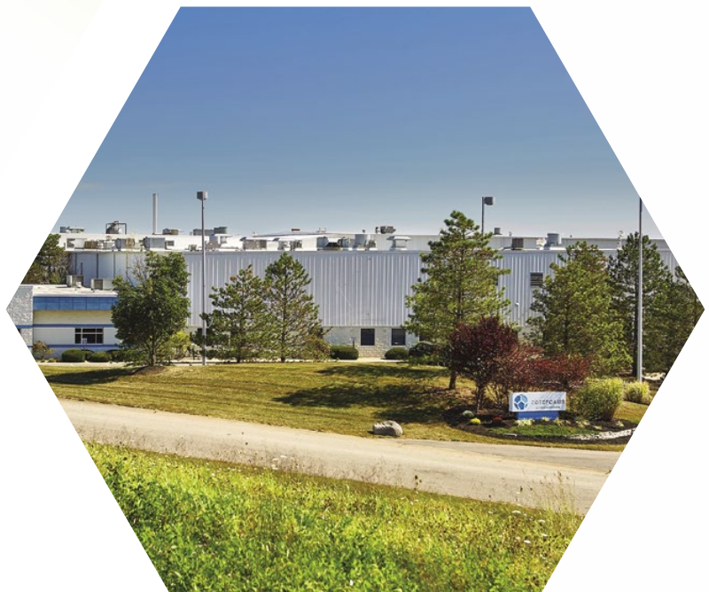
Foam manufacturing facility, Kentucky, USA
