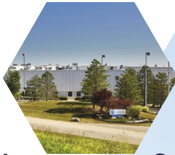
Foam manufacturing facility, Kentucky, USA
