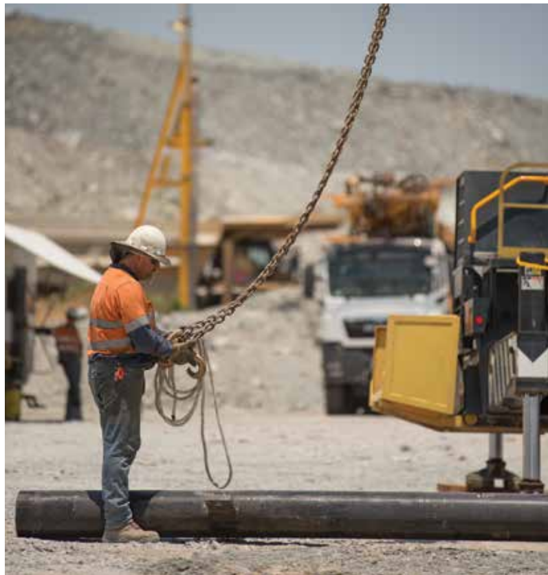
▲ Preparation work in Pit 3
