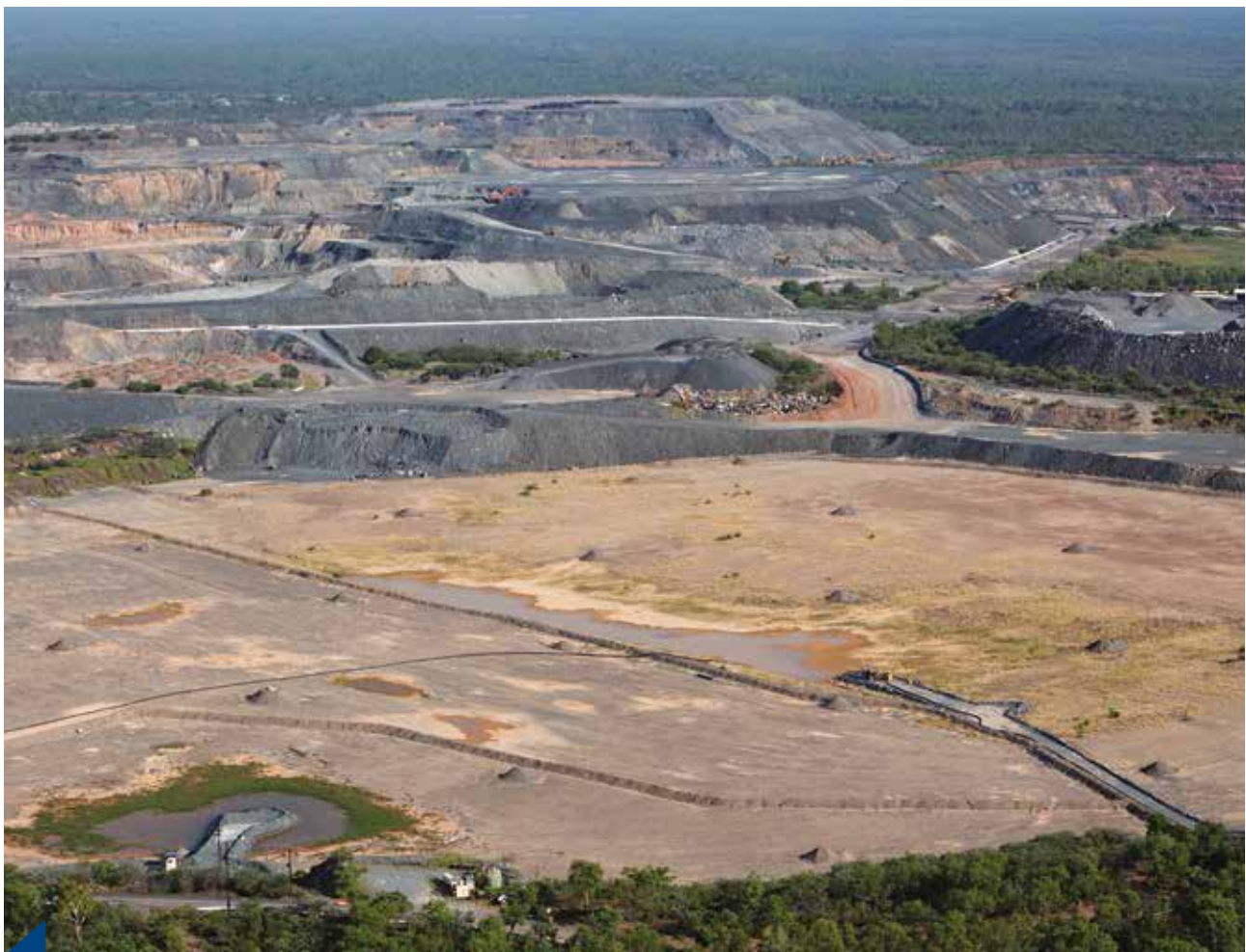
The capping of Pit 1 was completed in January 2016, the next stage of the rehabilitation process will be to commence bulk backfilling.
