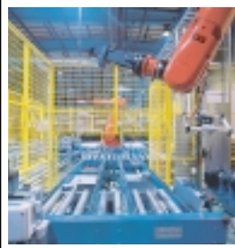
Powered Roller Conveyor
