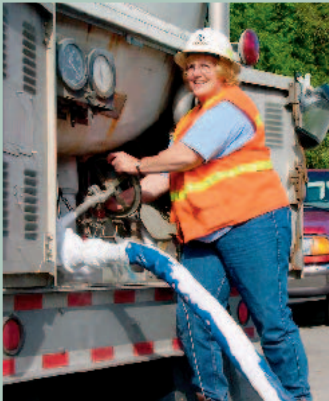
NW Natural sells liquefied natural gas to other local gas distributors to supplement their supplies. Above, Portland LNG Plant Operator Teri Carl adjusts the pressure that delivers LNG from the trailer into the ambient vaporizing unit. The vaporizer warms the LNG back into gaseous form for use in the distribution system.
