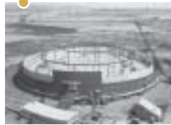
1969 Gasco's Linnton LNG tank is completed.
