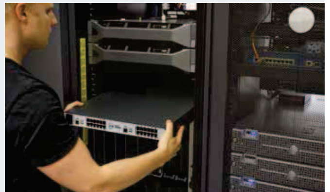
> TZ IXP Praetorian™ Junction installation.
