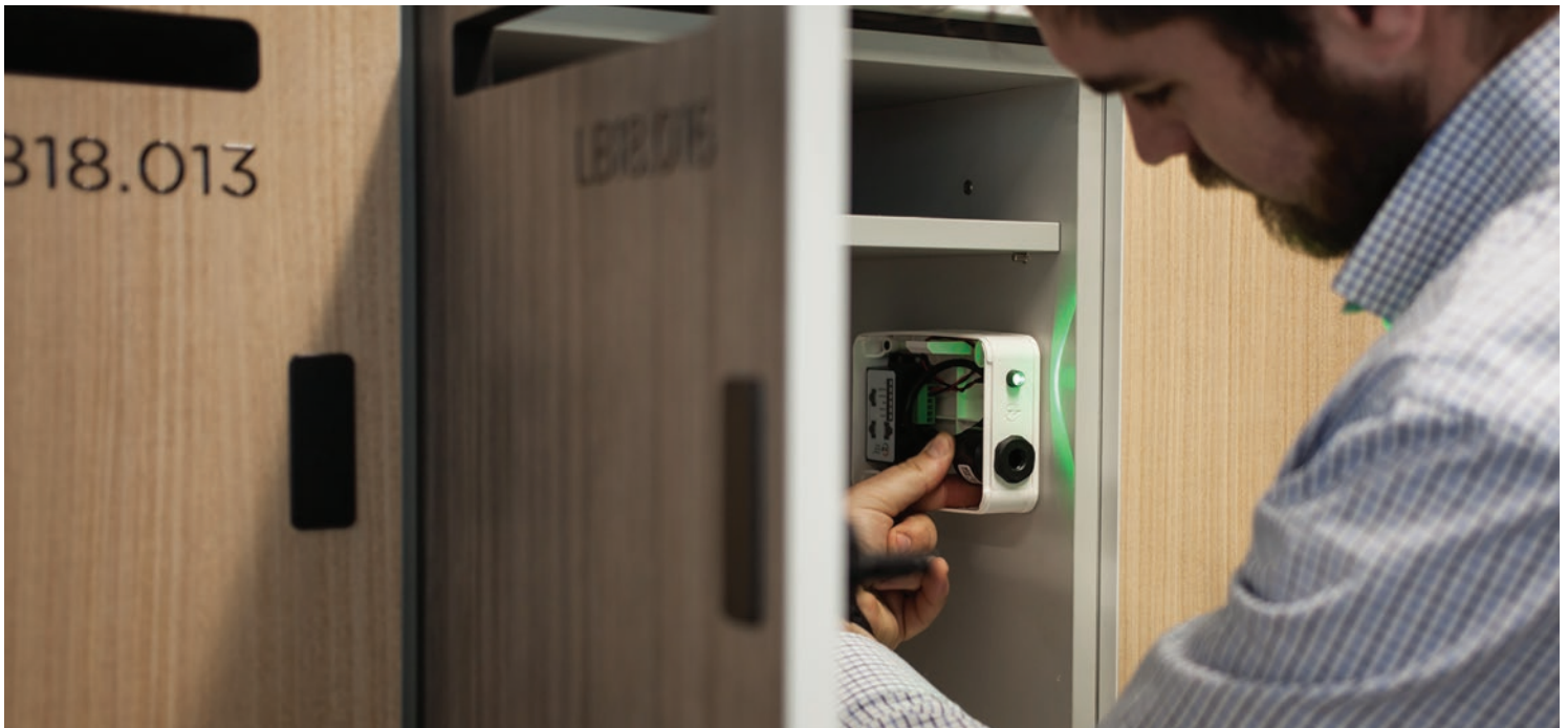
> Locker Install, Sydney Australia
