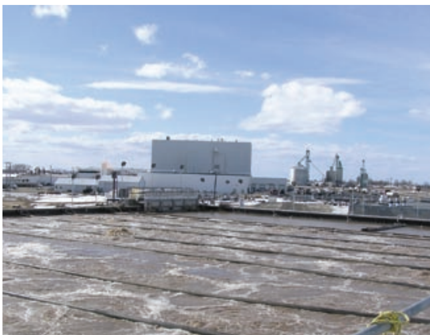
Waste water which is a by-product of milk processing is polished, stored and reused in plant boilers in Gooding.
