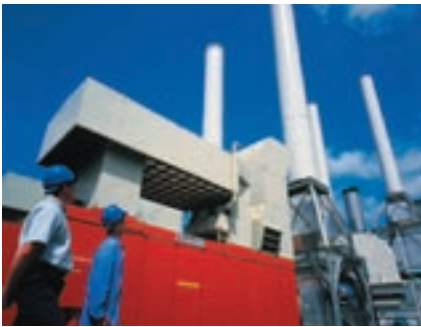
The combined heat and power plant at Ballyragget.
