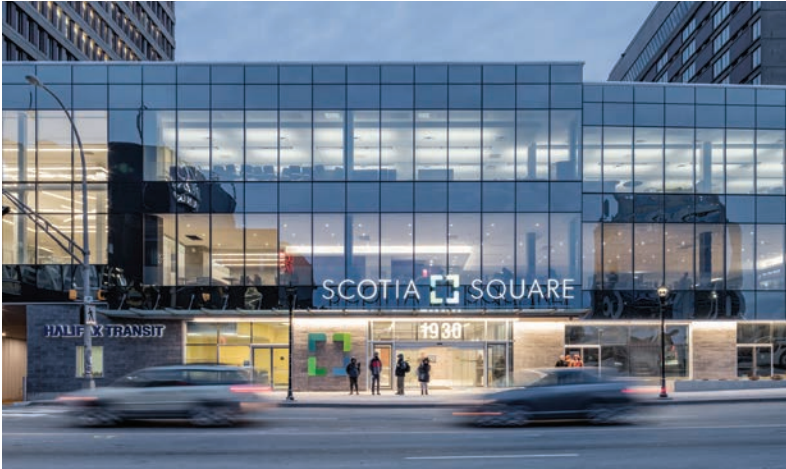
We began the process of greening our buildings at Scotia Square in 2008. Since then, completed projects have saved Crombie 18.6 million kWh of electricity and 22.5 million gallons of water per year, resulting in savings of over $2.5 million in annual operating costs.
