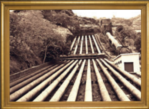
Pipelines to carry water to Power House
