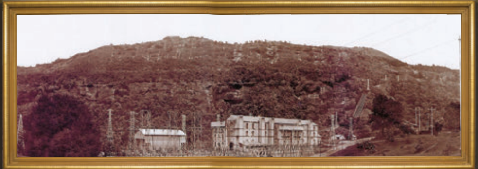
Khopoli Power House now called as Old Power House
