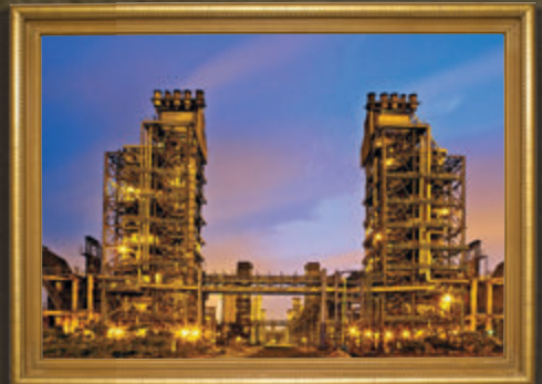
Haldia Power Station
