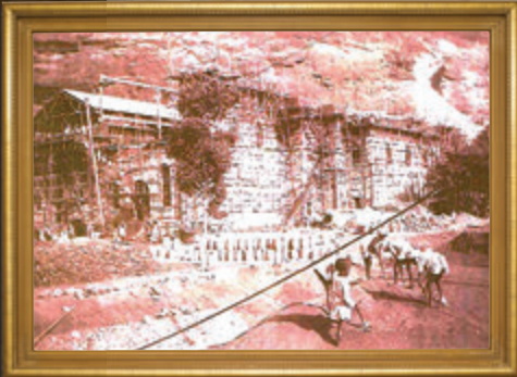
Construction at Khopoli Power House
