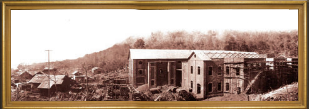
Old Power House under construction
