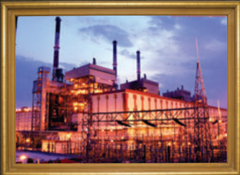
Jobbera Thermal Power Station
