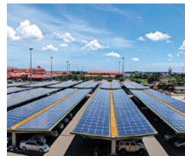
India's largest carport installation in Pune
