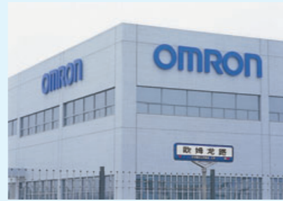
Production sites established and operated in Shanghai to produce sensors, FA systems, and control equipment
