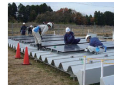
Solar system construction training
