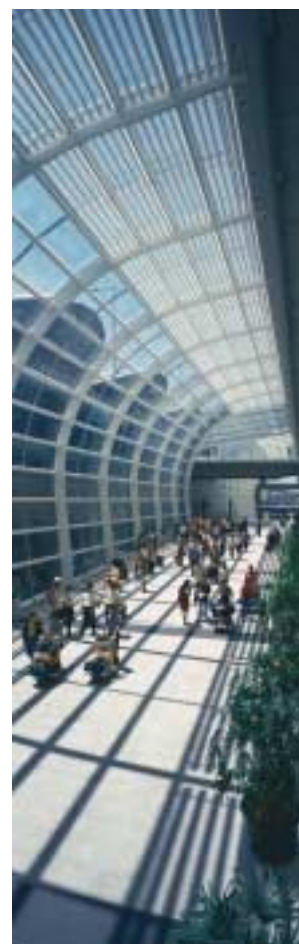
Memco elevator safety systems aid the swift movement of passengers through Hong Kong International Airport, China.
