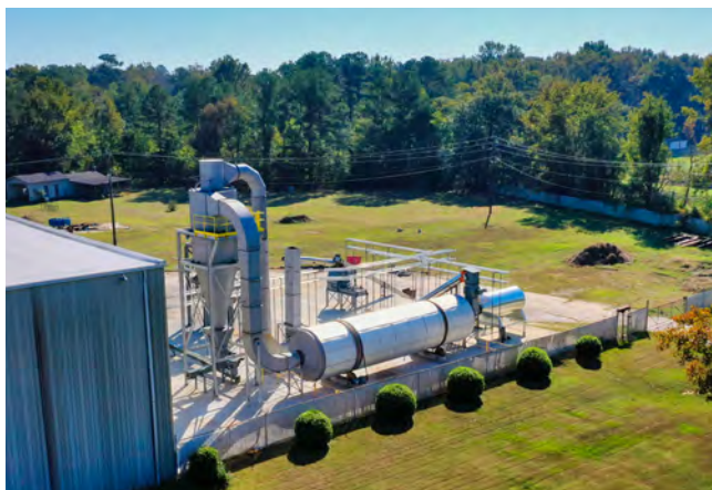
CoalSwitch® plant in construction at Lumberton.
