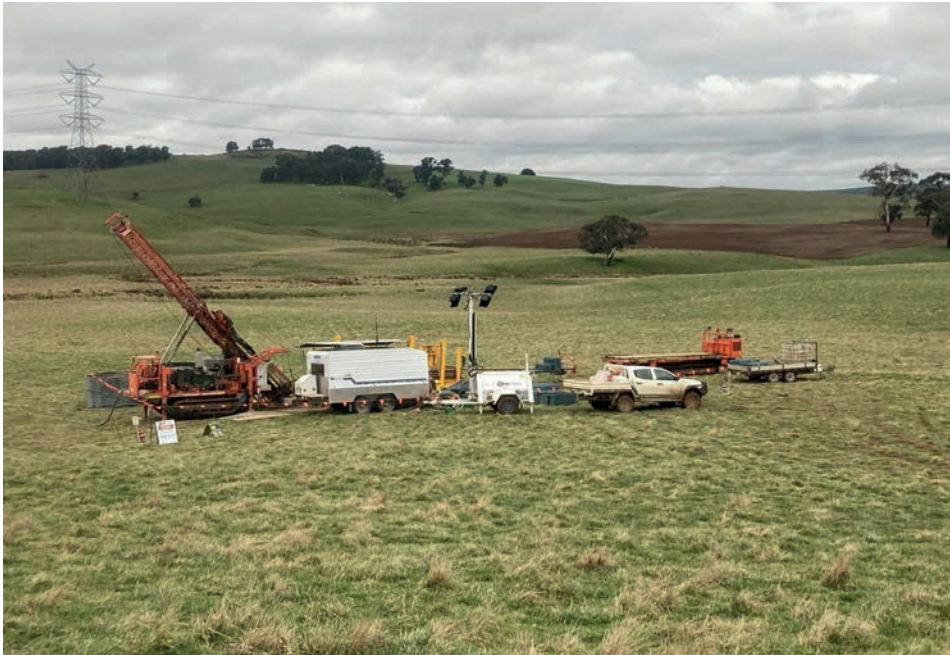
Photo 2 – Phase Two drilling underway at Bushranger
