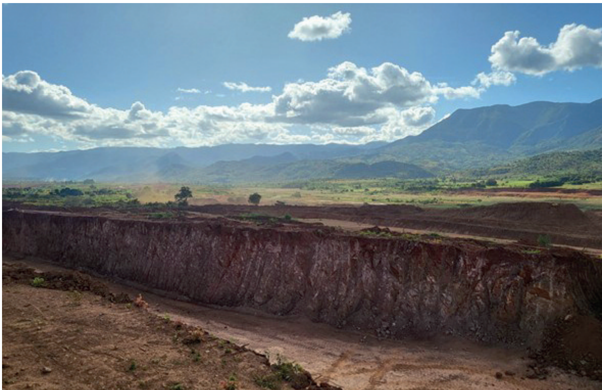
Photo 8 – Site works at Manica
