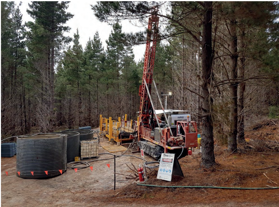
Photo 2 – Phase Two drilling progressing at Bushranger
