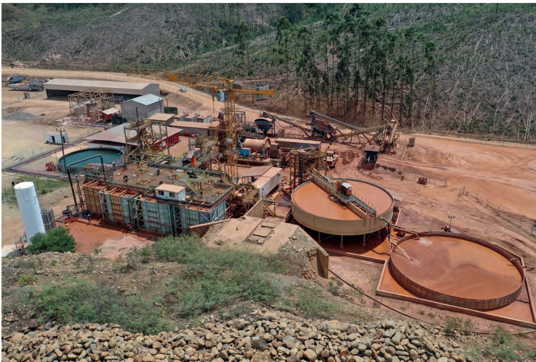
Photo 4 – The Manica Operation
