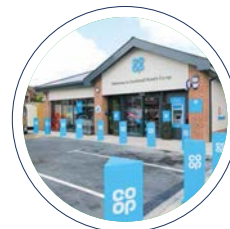
Apr 2017 Mansfield – Southwell Road West New build
