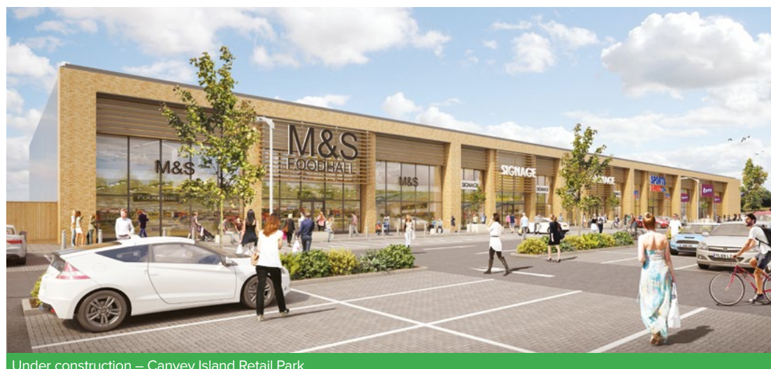
Under construction – Canvey Island Retail Park
