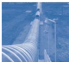
When completed, the over-land belt will move coal from the Warrior Slope to nearby preparation facilities.
