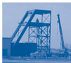
The headframe support structure is under construction at the Dotiki mine.
