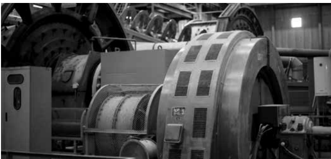
c.15.5Mtpa of plant processing capacity
