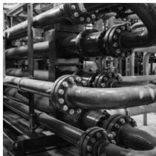
POX Hub staged commissioning scheduled from Q4 2018
