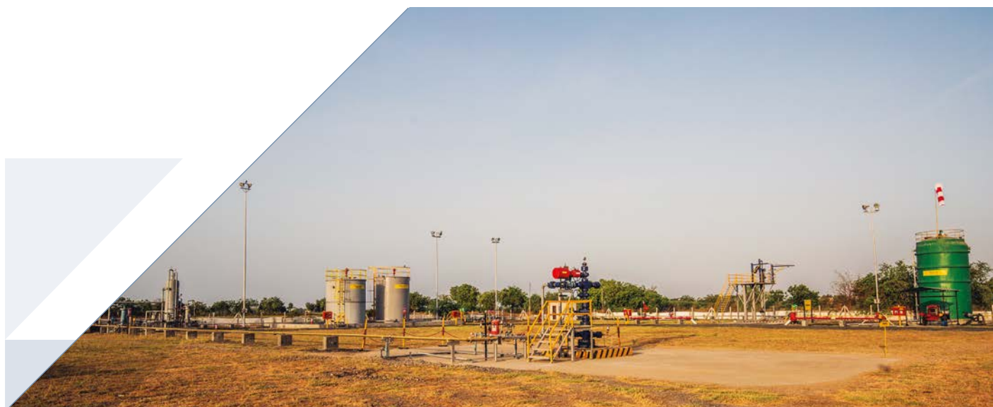
Figure 4: Cambay-73 Production Facility
