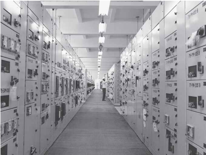
L&T's custom-engineered switchboards, equipped with both conventional and 'intelligent' protection, control and communication systems meet the power control and distribution needs of industry.
