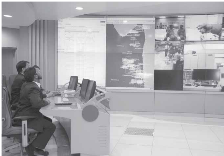
Supervisory Control And Data Acquisition system designed, supplied and commissioned by L&T for Onshore Control Centres (OCCs) for offshore operations of Oil & Natural Gas Corporation. The system connects 133 wellhead platforms, 13 process complexes and nine drilling rigs to OCC.
