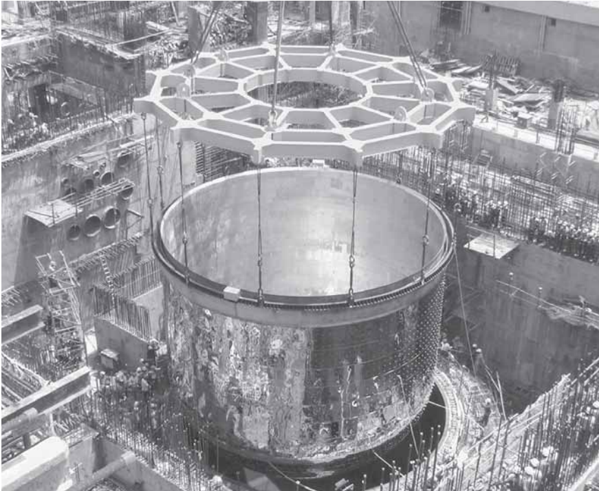
Reactor vessel for Fast Breeder Reactor (FBR) being lowered into a vault. The mirror-polished thermal insulation panel increases the effectiveness of the vessel. L&T is at the forefront of India's FBR programme.
