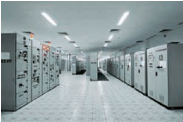
L&T's custom-engineered switchboards are equipped with both conventional and intelligent protection, control and communication systems.
