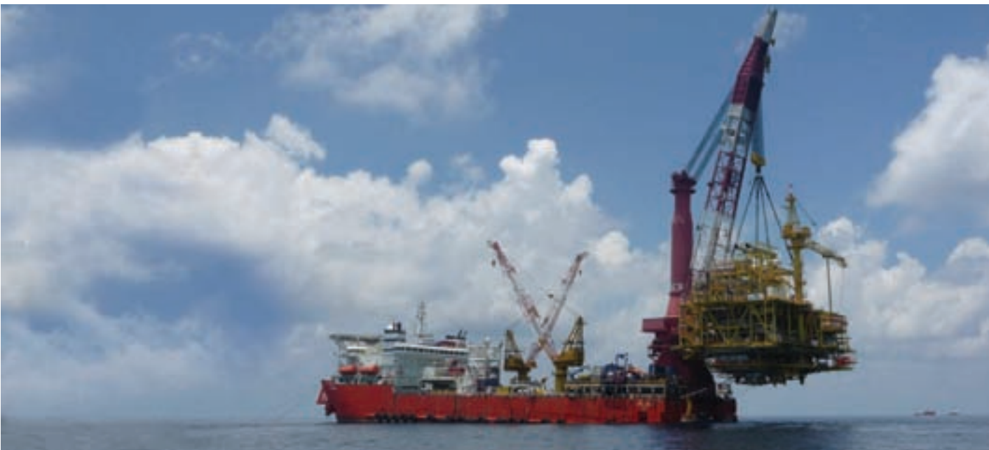
L&T's heavy-lift-cum-pipelay vessel LTS 3000 installing a topside for Newfield Peninsula in Malaysia.
