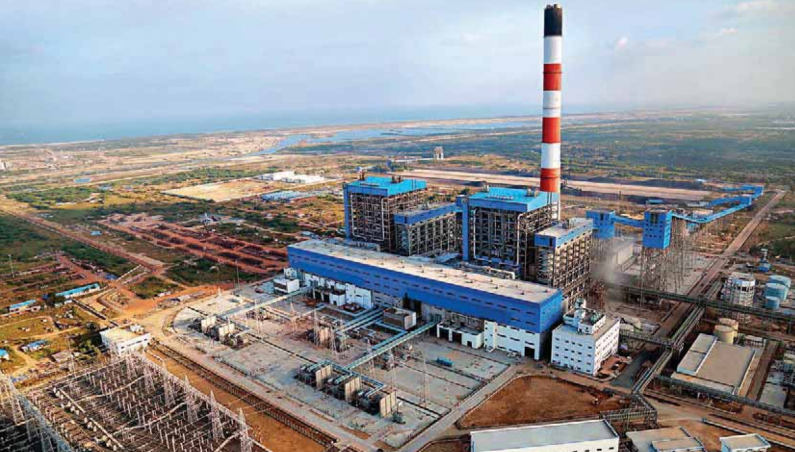
2x800 MW supercritical thermal power plant at Krishnapatam, Andhra Pradesh. L&T has manufactured critical equipment for supercritical power plants across India.
