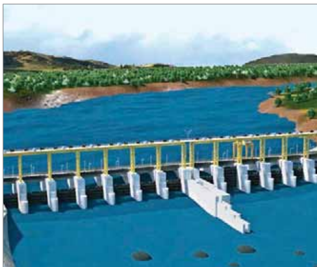
The barrage being built on the Kharkai river in Eastern India.
