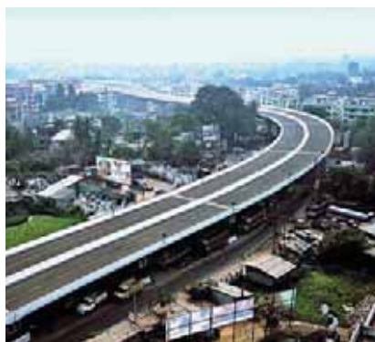
A flyover built by L&T.
