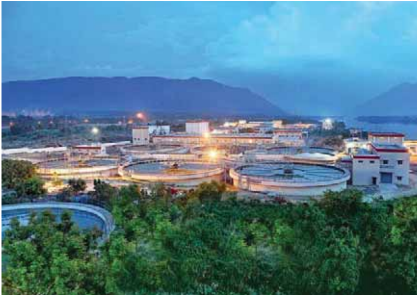
Water-treatment plant for Vellore Water Supply Scheme, Tamil Nadu.
