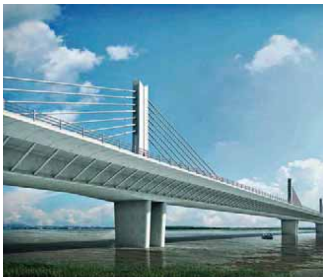
The majestic 9.76-km Kachi Dargah Bridge across the mighty Ganga in Bihar will be India’s longest extradosed bridge.
