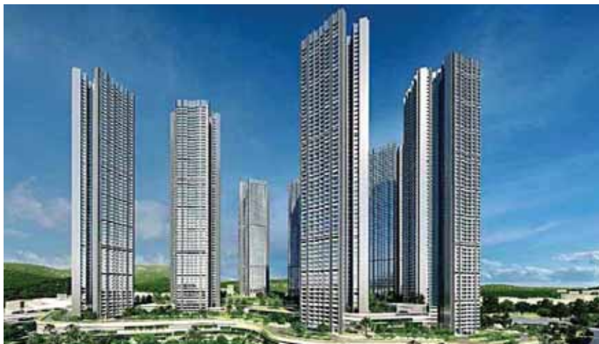
Oberoi Sky City at Borivali, Mumbai. L&T builds elite, mass and affordable housing complexes on a turnkey basis.
