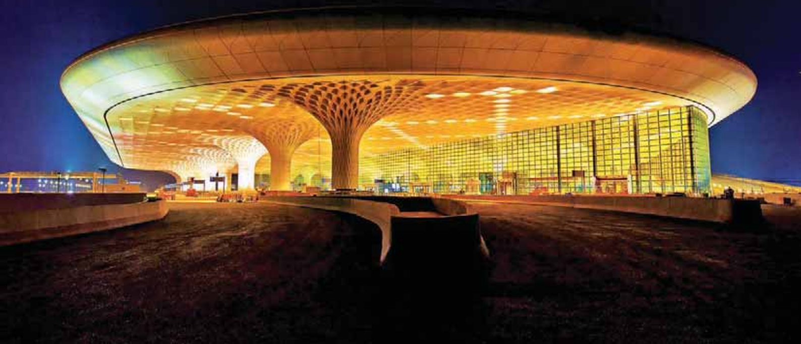
Terminal 2, Mumbai International Airport - an iconic structure which integrates world-class design, architecture and operational efficiency. L&T has built several airports in India and in the Middle East.
