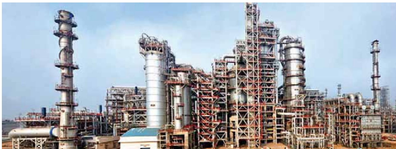
FCC reactor regenerator section for IOCL at its Paradip Refinery.
