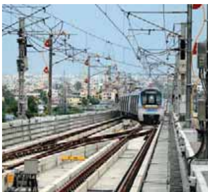
Metro electrification & signaling project.
