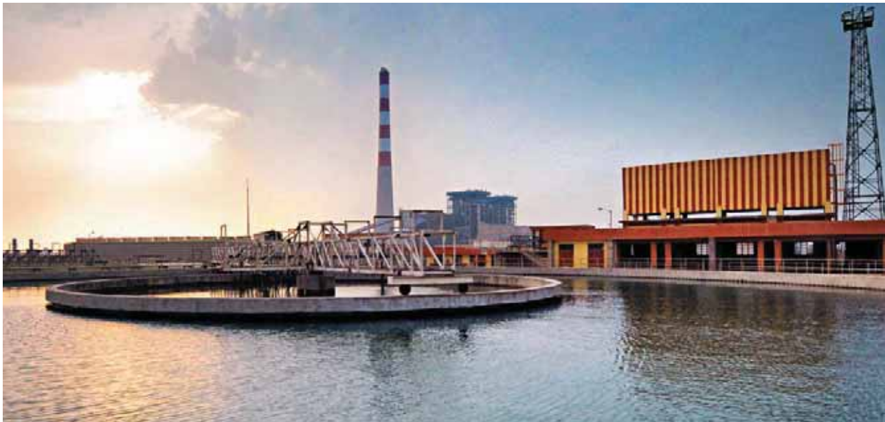
Water pre-treatment plant for a power plant in Sagardighi, West Bengal.
