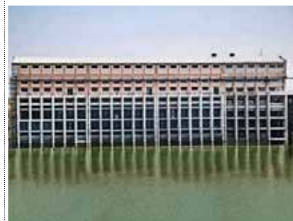
Hanamapur Lift Irrigation Project, Karnataka.
