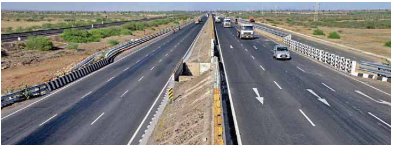
The 56.17-km six-lane stretch of NH 8A between Samakhiali and Gandhidham in Gujarat connects the important port towns of Kandla and Mundra to north India.
