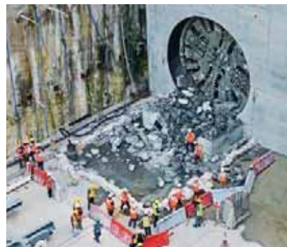
Tunnel-boring on the Doha Metro.
