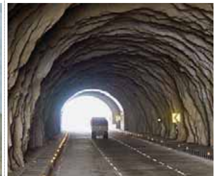
Tunnel on the Beawar-Pali-Pindwara road project.
