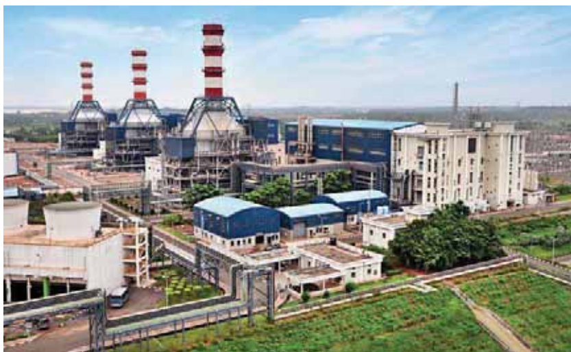
Natural-gas-fired combined-cycle power plant built by L&T at Vemagiri in Andhra Pradesh.
