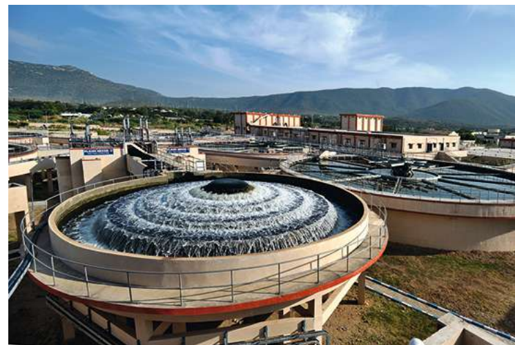
181 MLD water treatment plant for Vellore Water Supply scheme.
