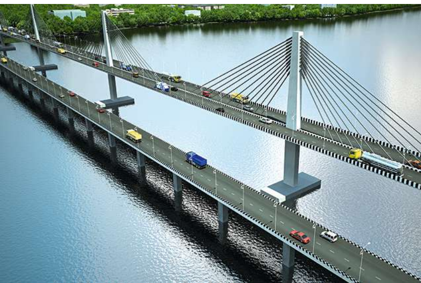
Across River Mandovi in Goa, L&T is building one of India's longest cable-stayed bridges.
