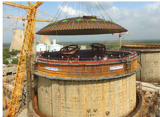
Dome erection at the Kakrapar Atomic Power project, Gujarat
