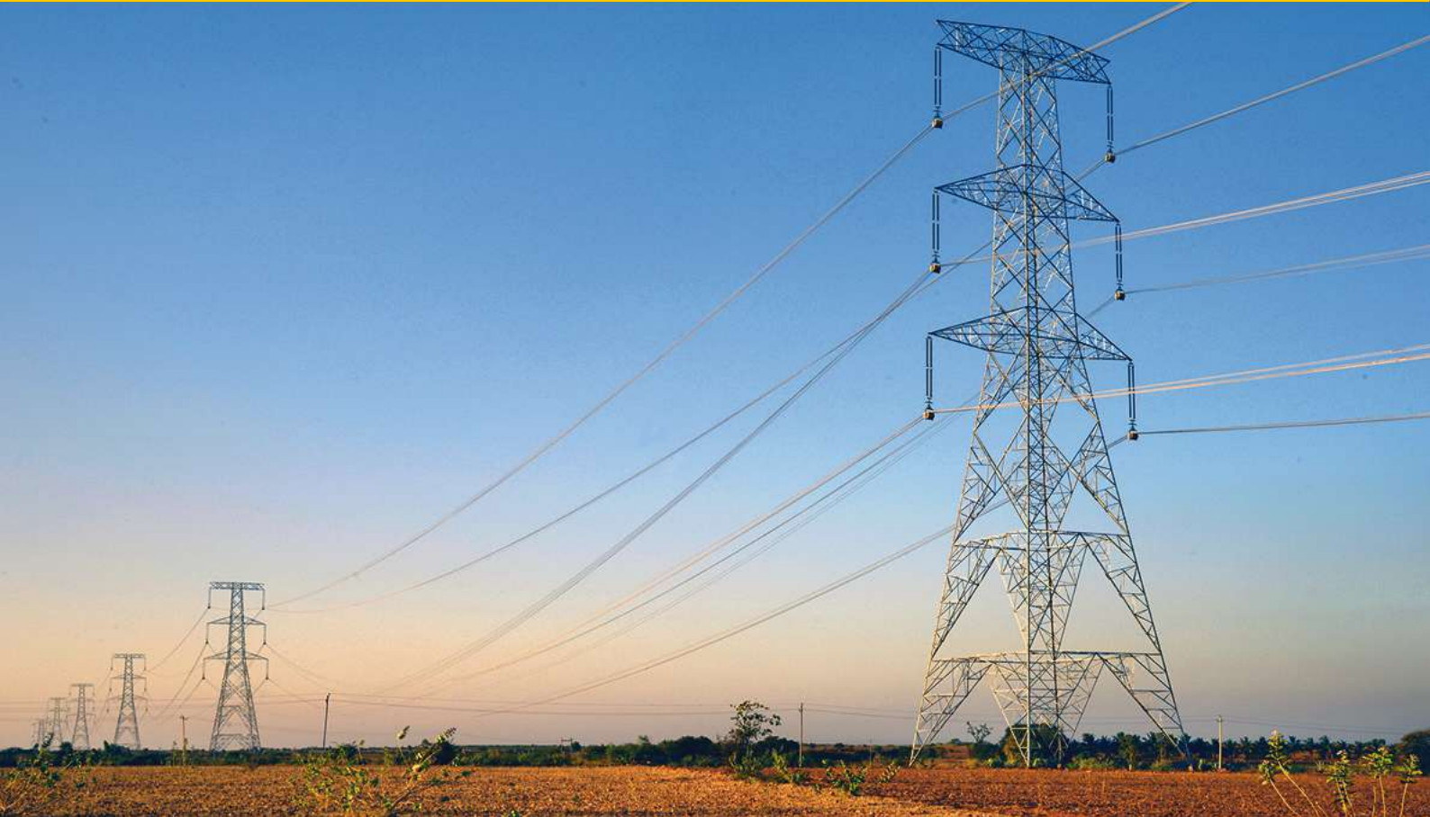
Kudgi Power Transmission Line project, Karnataka.
