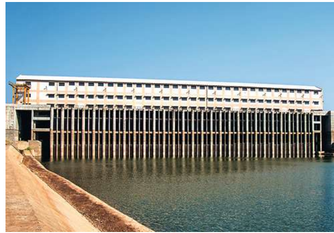
Hanamapur lift irrigation project, Karnataka.
