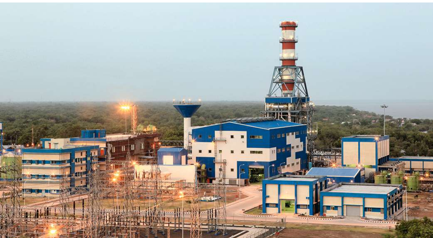
On EPC basis, L&T undertook the 375 MW single-shaft combined cycle power plant project for Gujarat State Electricity Corporation at Dhuvaran in Gujarat.
