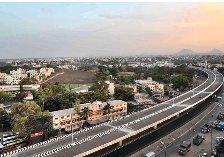
An Elevated Corridor sweeping over a city – one of L&T's many road development projects.
