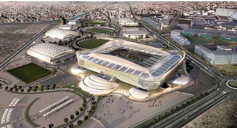
Artist's impression of football stadium being built in Qatar, incorporating design and processes to minimize environmental impact
