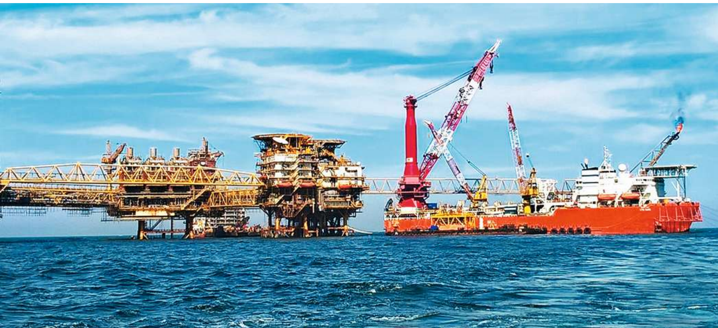
Additional development of Vasai East Project for ONGC. The scope included EPCIC of 2 wellhead platforms, 35 km pipelines and modification.
