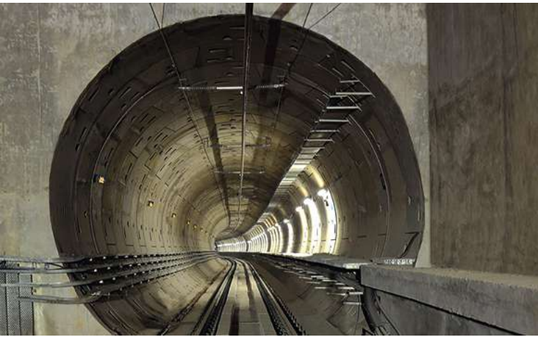
An underground section of the Chennai Metro.
