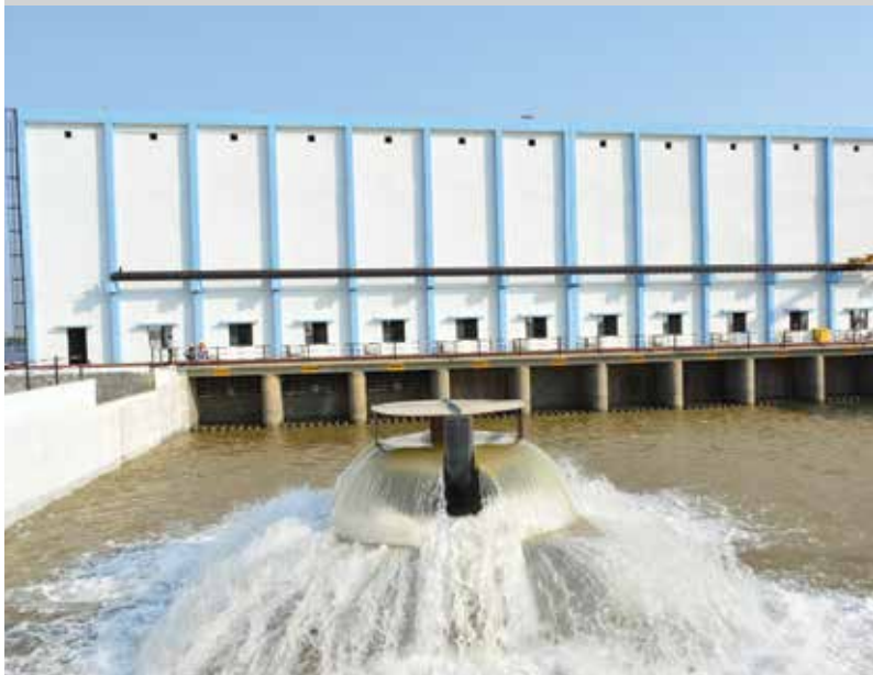
Sauni Yojana Lift Irrigation Project, Gujarat
