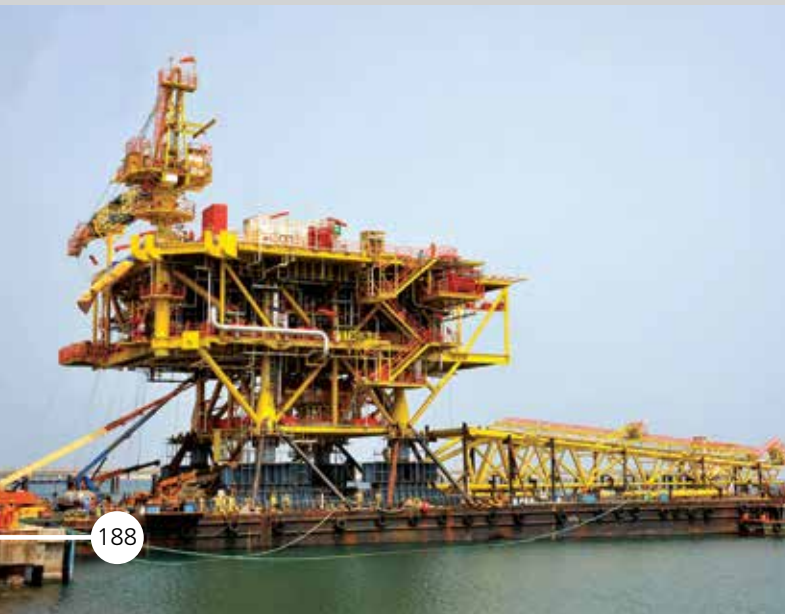
Sailing out of Wellhead Platform Topside from Kattupalli Facility
