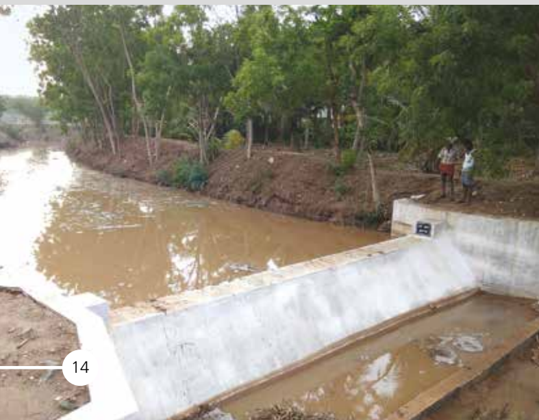
Water conservation structures built to meet domestic needs, Chettipalayam, Tamil Nadu.
