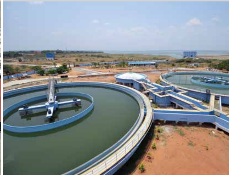
Medak & Sangareddy Water Supply Project, Telangana
