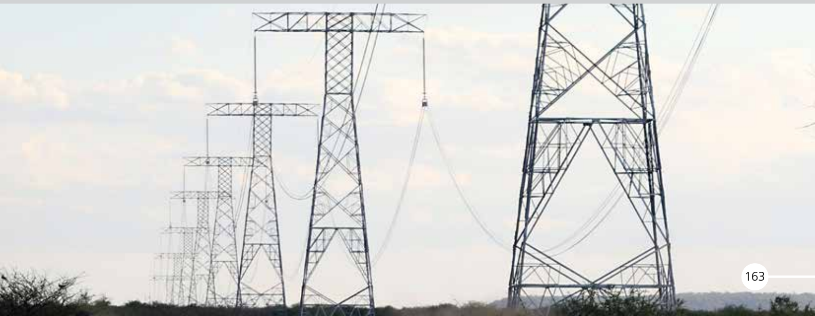
500kV HVDC Transmission Line at Kenya
