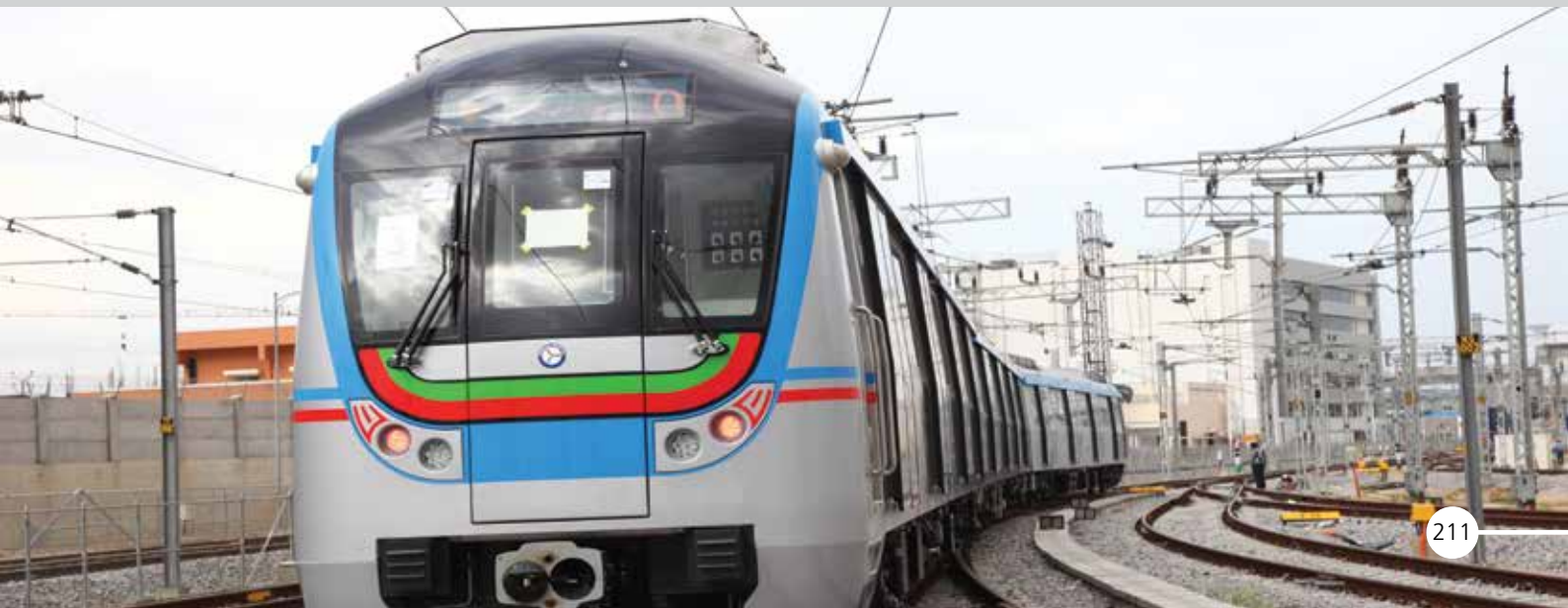
Hyderabad Metro Rail project
