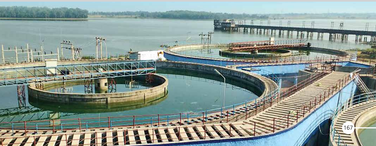
114 MLD Water Treatment Plant at Ranchi, Jharkhand
