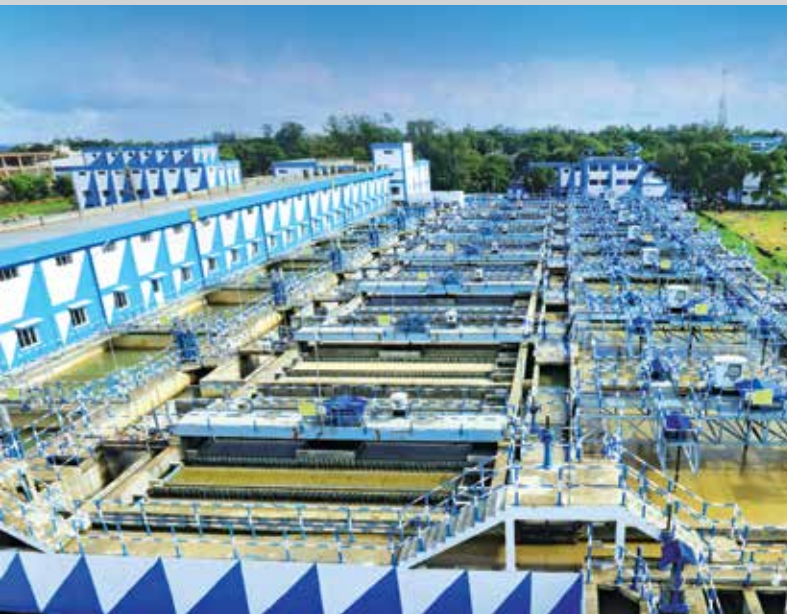
227 MLD Water Treatment Plant at Garden Reach, Kolkata, West Bengal
