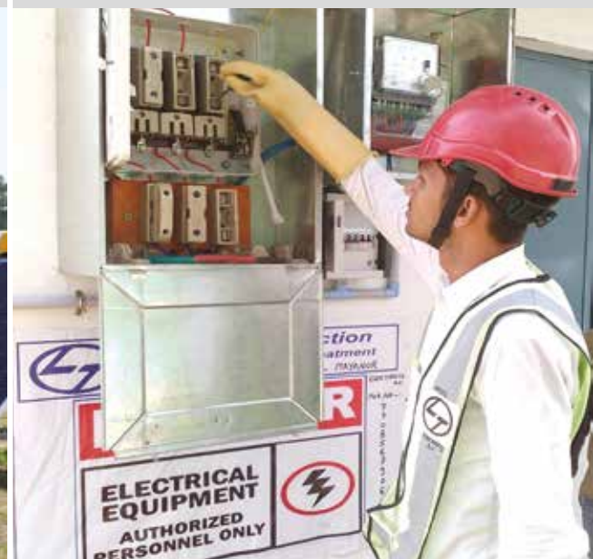
CSTI-trained Electrician working at Dindigul project
