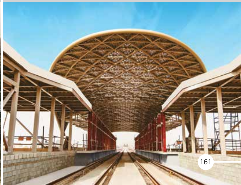
Canopy erected for a station building at Riyadh Metro
