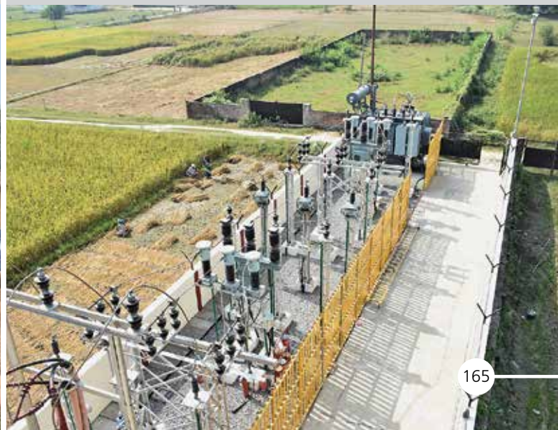
Restructured Accelerated Power Development & Reforms Programme, Varanasi
