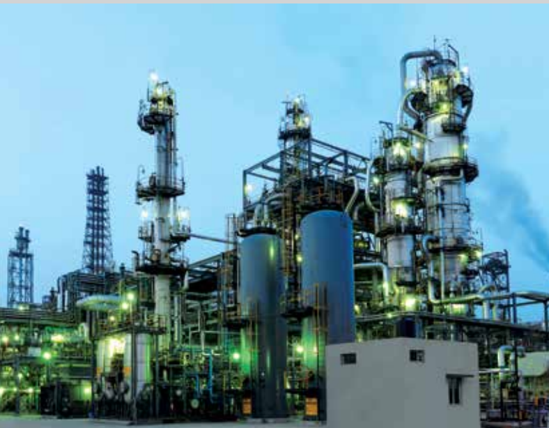
900 TPD ammonia plant of National Fertilizers Limited, Panipat.
