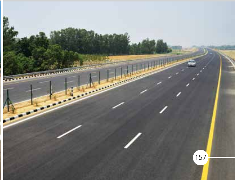
Six-lane Access Controlled Expressway from Unnao to Lucknow
