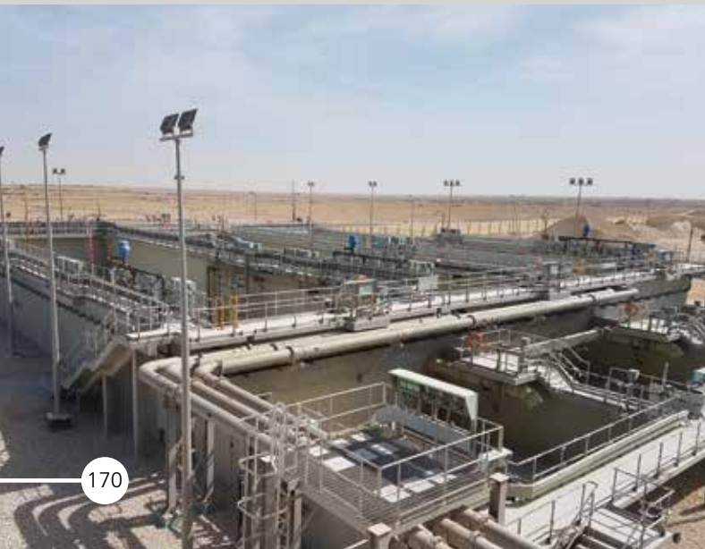
Sewage Treatment Plant at Al Shamal, Qatar
