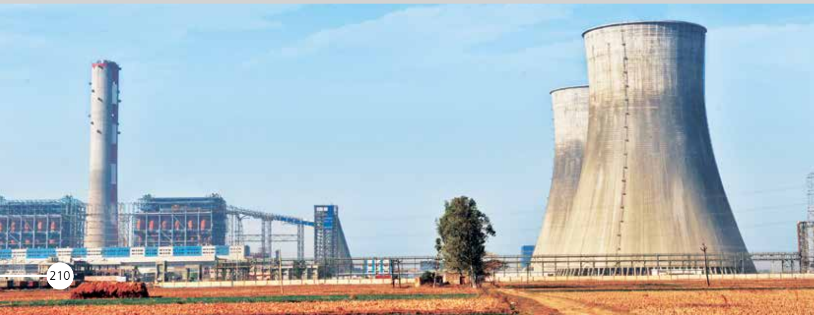
Rajpura Supercritical Thermal Power Plant
