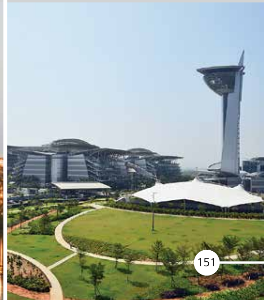
TCS Customer Care Centre, Chennai
