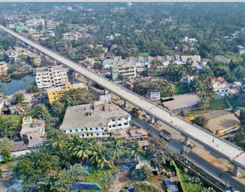
7.4 km Elevated Corridor at Bhatnagar Kolkata
