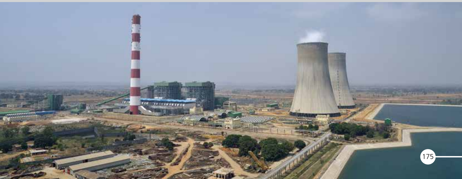
2x660 MW Supercritical Thermal Power Plant at Nigra in Singrauli district, Madhya Pradesh. L&T executed Boiler and Turbine Island on EPC basis.
