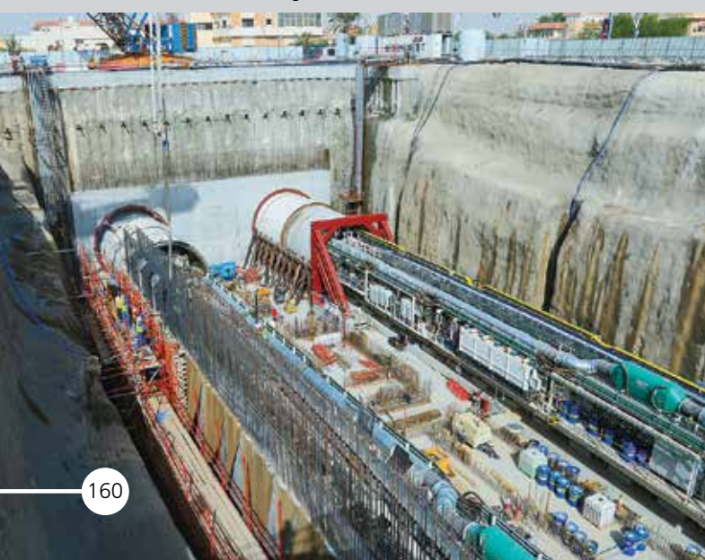
One of the station buildings under construction for Doha Metro, Qatar
