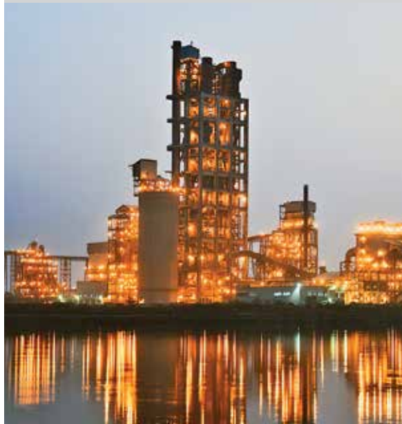
Orient Cement project at Chittapur in Hyderabad
