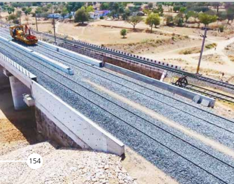
A completed section of Western Dedicated Freight Corridor - Civil & Trackwork
