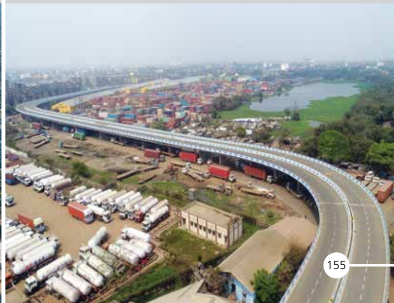
Garden Reach Flyover at Kolkata
