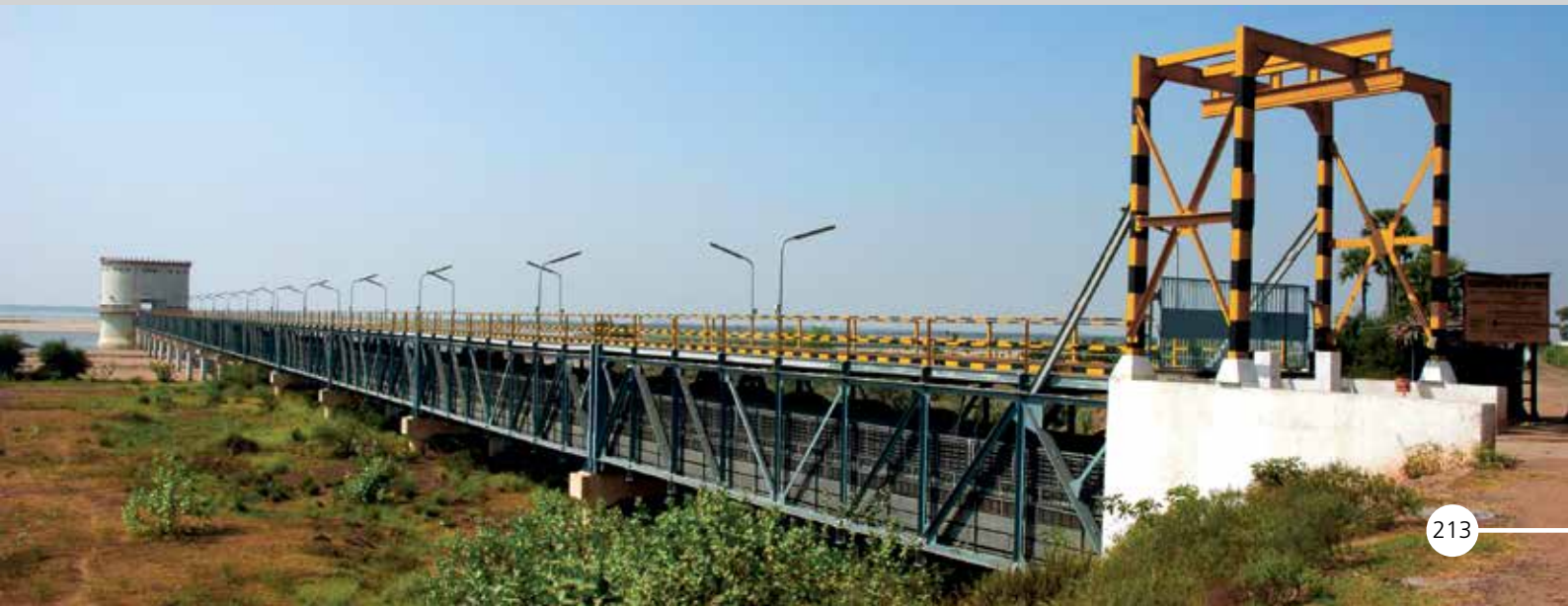
Visakhapatnam industrial water supply project, Andra Pradesh
