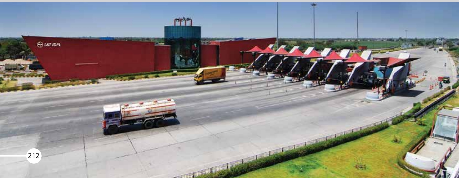
Vadodara-Bharuch Toll plaza, Gujarat
