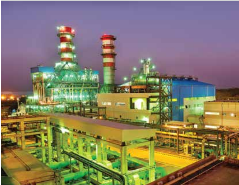
225 MW Combined Cycle Power Plant, Sikalbaha, Bangladesh, built on EPC basis
