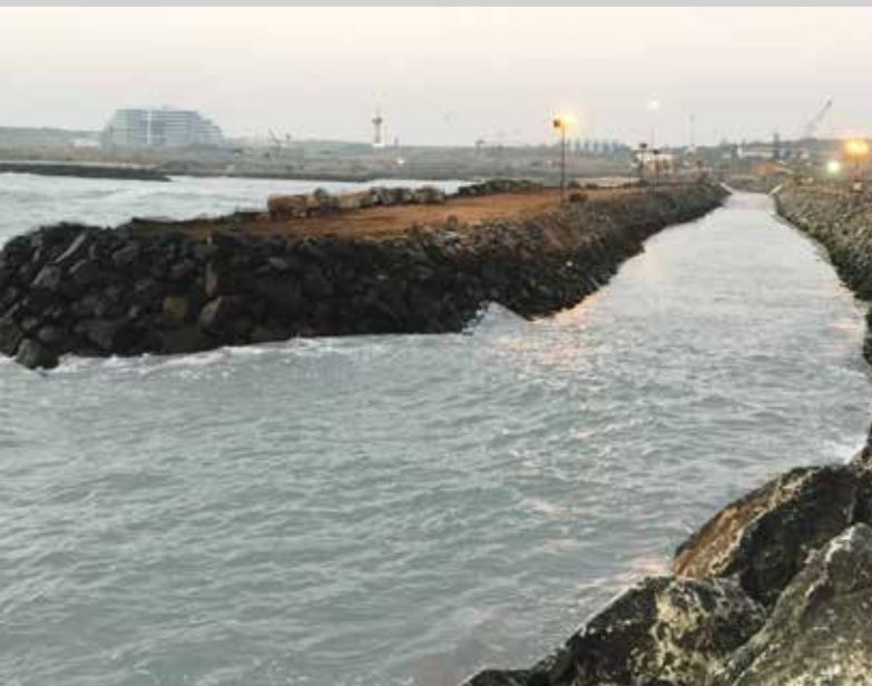
Break Water construction at Kudankulam Nuclear Project
