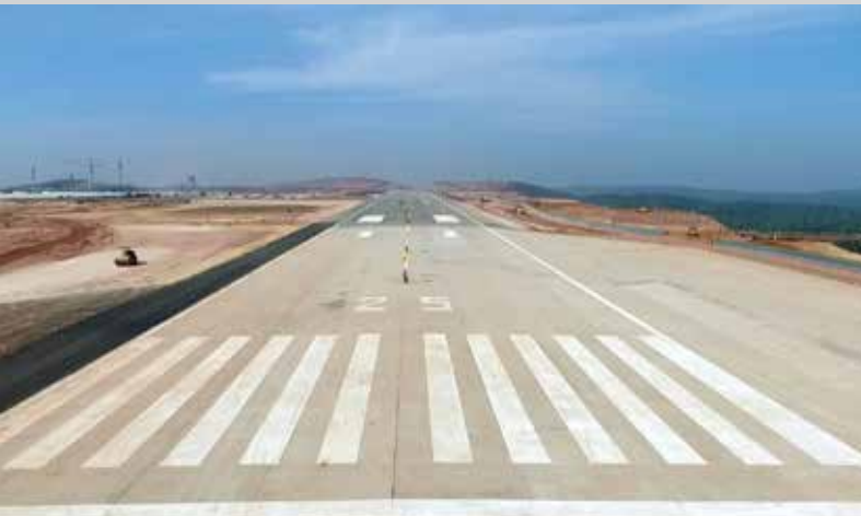
Kannur International Airport Runway
