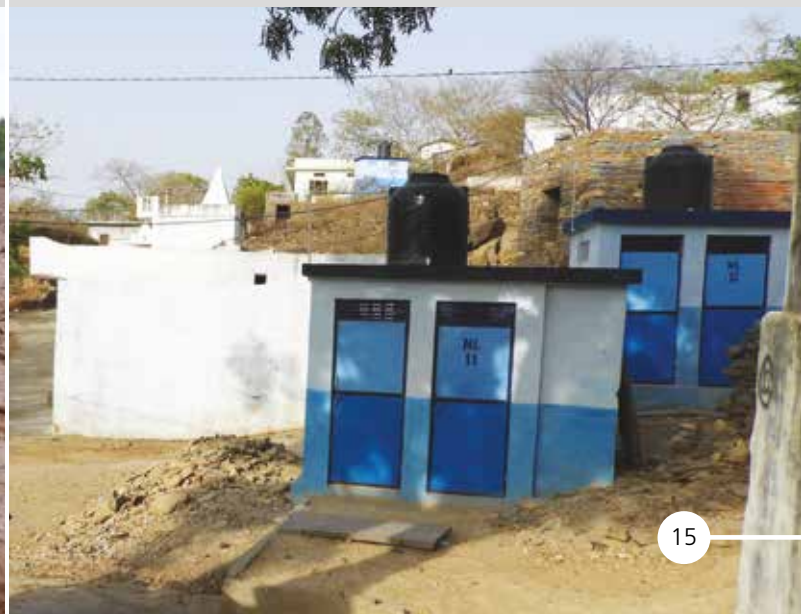
Toilet Blocks at Lasadiya, Bhim, Rajasthan
