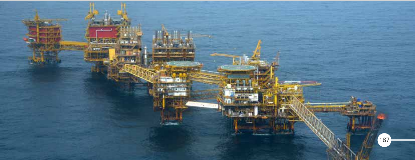
Bassein Development Project for ONGC including platforms (Living Quarters & BH Wellhead), pipelines, bridges and modifications
