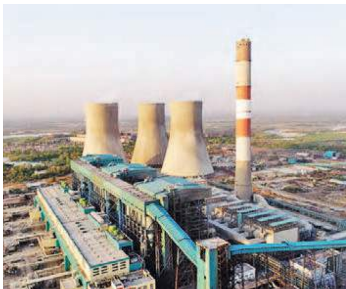
3x660 MW Koradi Thermal Power Plant, Maharashtra
