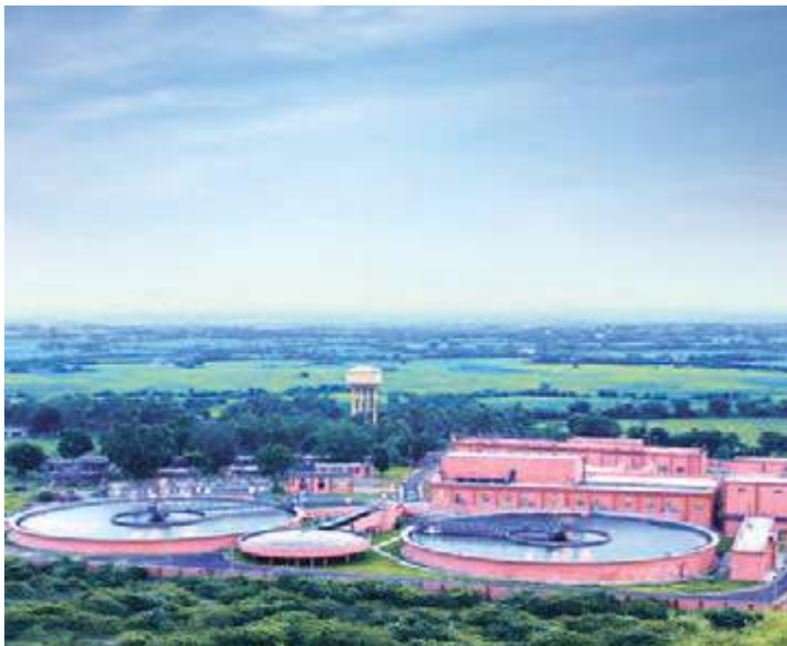
74 MLD Water Treatment Plant at Bisalpur Tonk Unniyara
