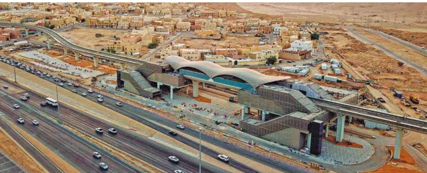
Riyadh Metro - L&T is building metro networks in India and select geographies
