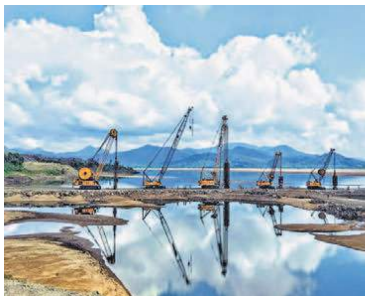
Cut-off-wall, Polavaram Dam, Andhra Pradesh
