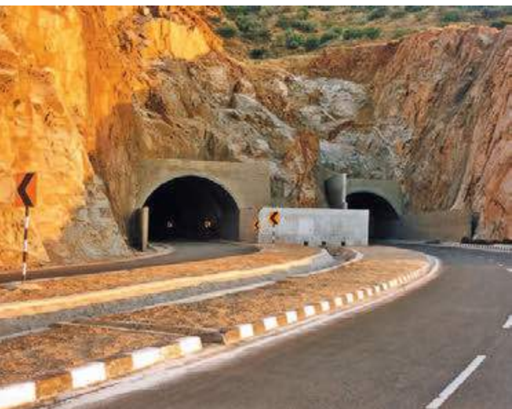
The 221.4 km Beawar – Pali – Pindwara road in Rajasthan is the longest four lane road project developed under the (PPP) model in the National Highways sector.
