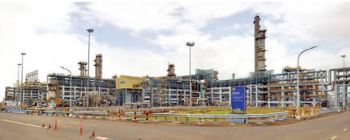
Construction of the world's largest ethylene cracker (1.4 MMTPA) for Reliance Industries, Jamnagar, India
