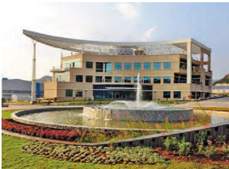
L&T's green portfolio includes green buildings and a large number of eco-friendly products, systems and solutions.
