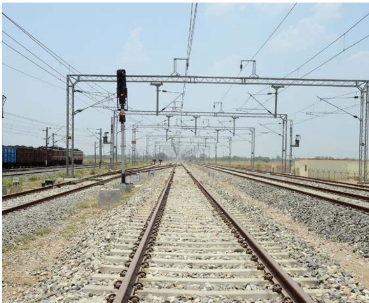
Railway electrification by L&T on Eastern Dedicated Freight Corridor
