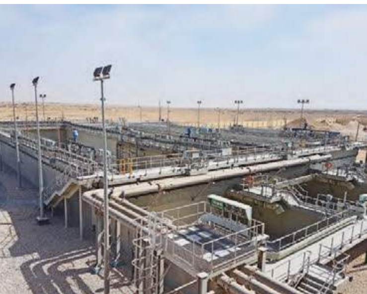
Al Shammal Water Treatment Plant at Qatar
