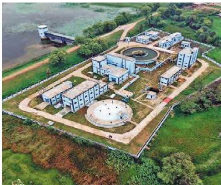
10.6 MLD Water Treatment Plant, Bagidora
