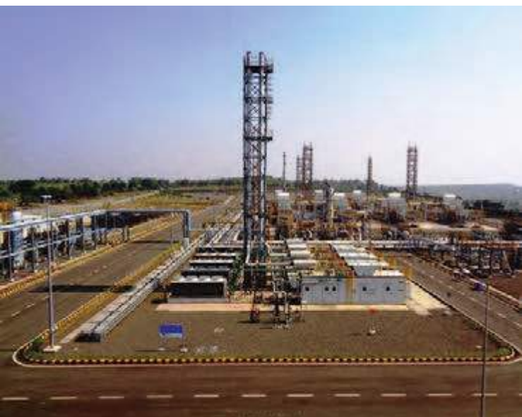
Group Gathering Station-11 for RIL's Coal Bed Methane Field Development Project, Shahdol, Madhya Pradesh
