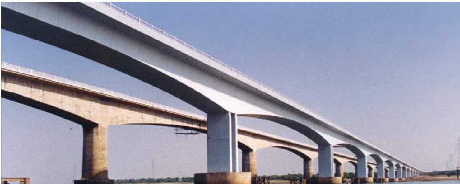
India's longest extra-dosed, cable stayed bridge over the Narmada, Gujarat
