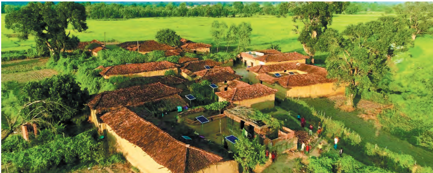
Micro Grid Project for rural electrification, Bihar
