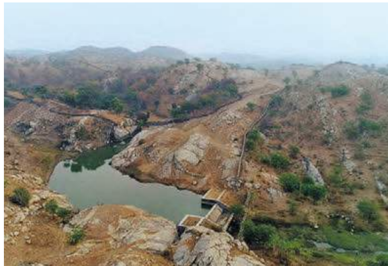
Rainwater harvesting through an anicut, at Village Kemriya, Bhim Block, Rajasthan
