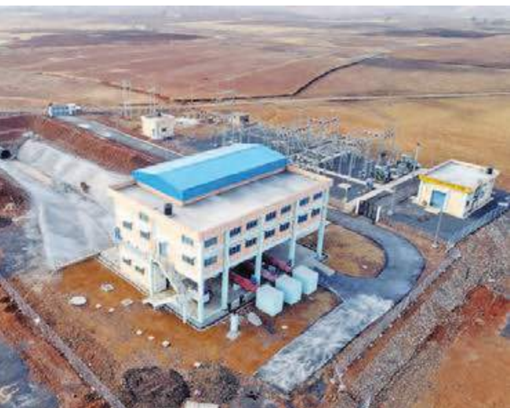
Pump house for Mohanpura Lift Irrigation Scheme
