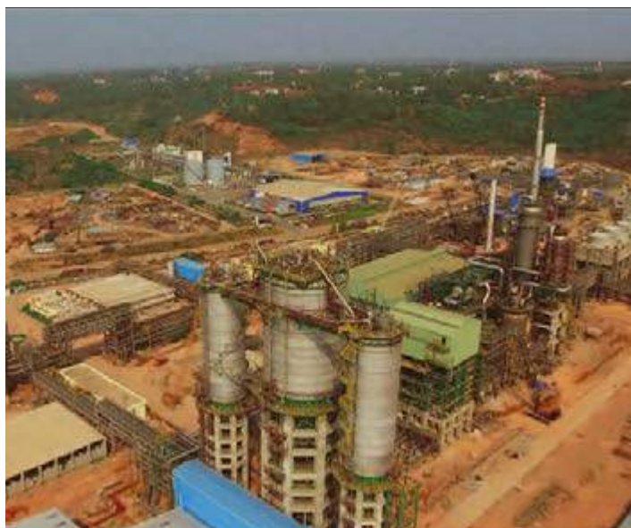
Panoramic view of PTA Plant for JBF Industries, Mangalore
