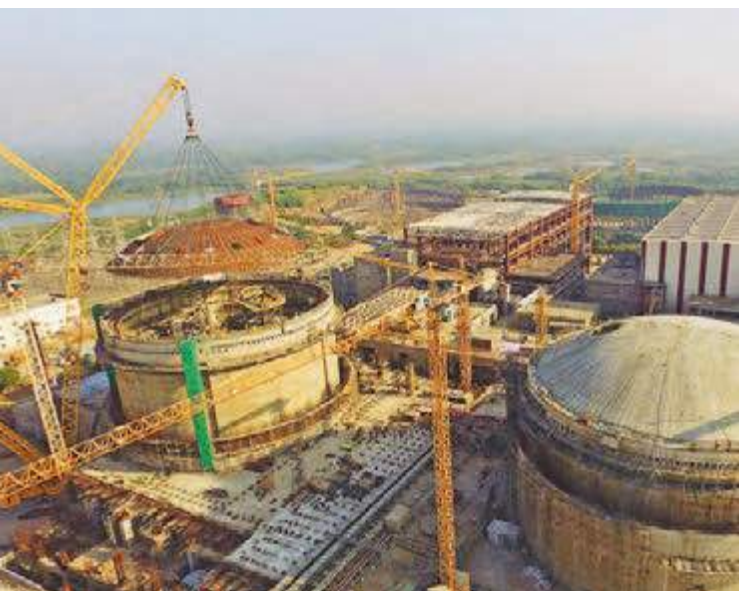
Kakrapar Atomic Power Plant, Gujarat, under construction
