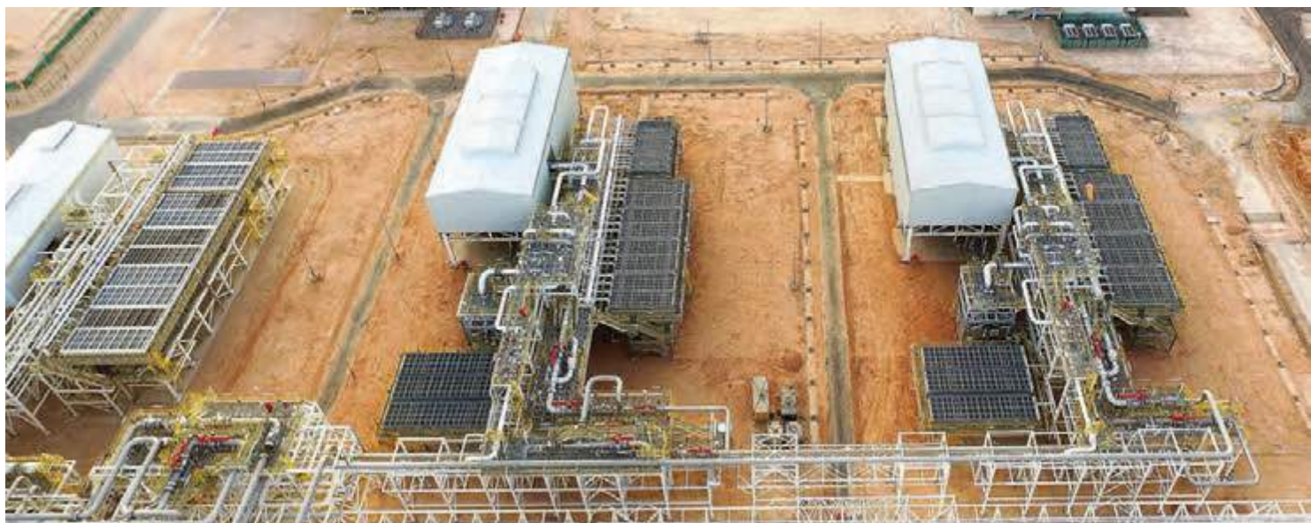
Saih Nihaydah Gas Compression Project (SNDC2) for Petroleum Development Oman (PDO)
