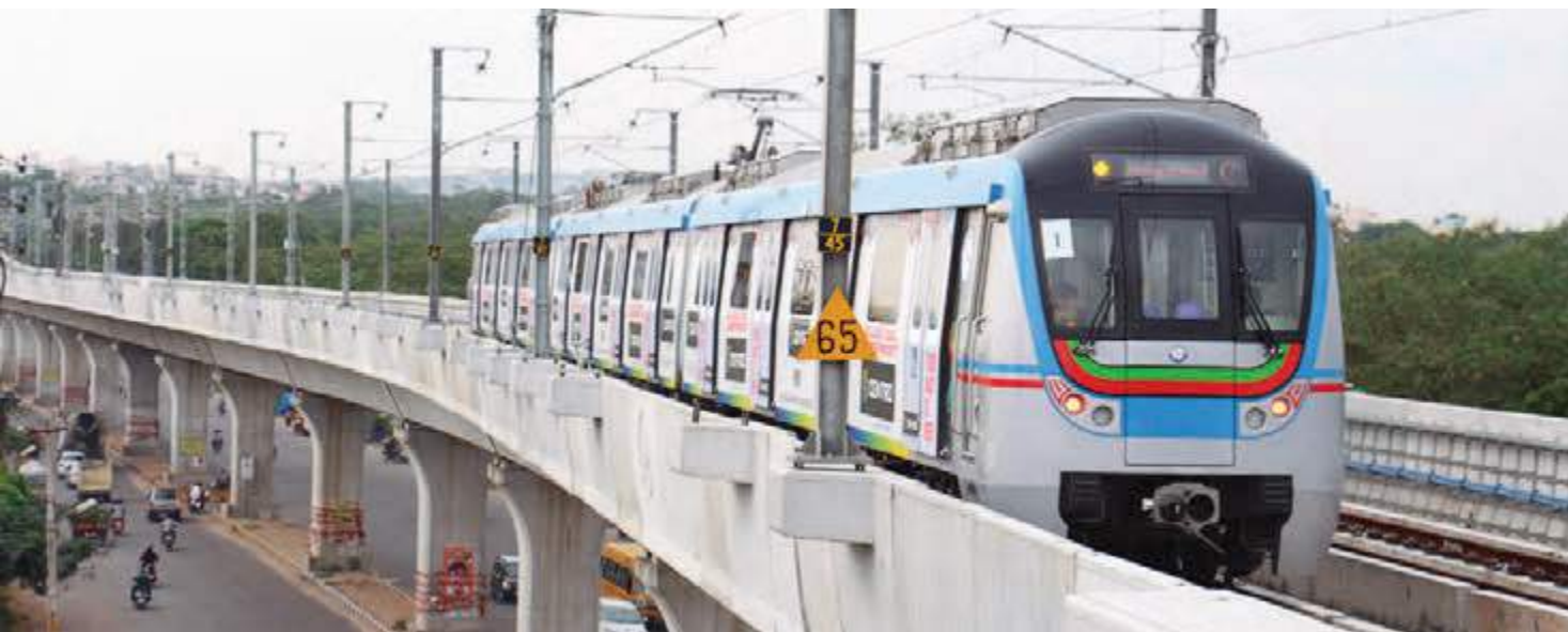
A section of the Hyderabad Metro
