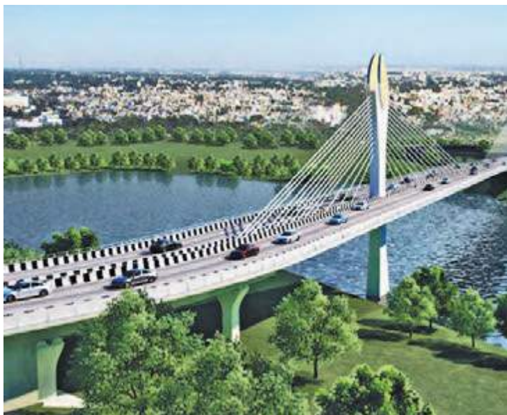
Cable-stayed bridge across Durgam Cheruvu Lake, Telangana
