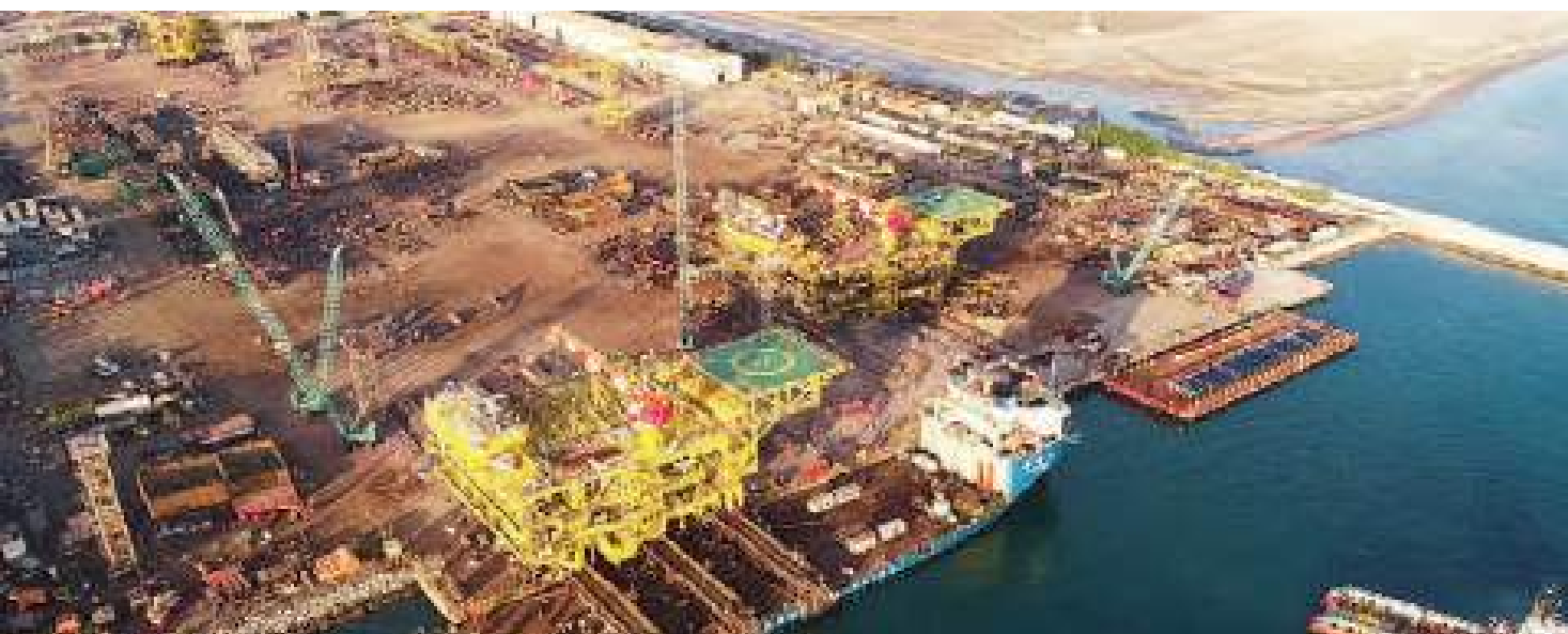
Load-out of two mega Tie-in Platforms (7000 MT each) for Hasbah Field, Saudi Aramco from L&T Hydrocarbon Engineering's Oman facility
