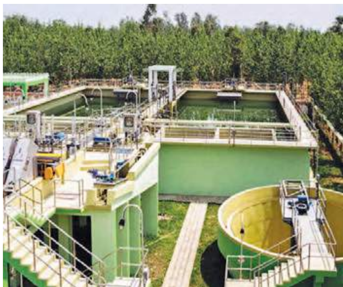
Sewage Treatment Plant at Rampur
