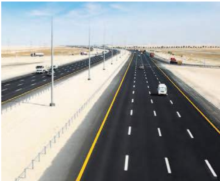
Mafrag-Ghweifat Highway, Abu Dhabi
