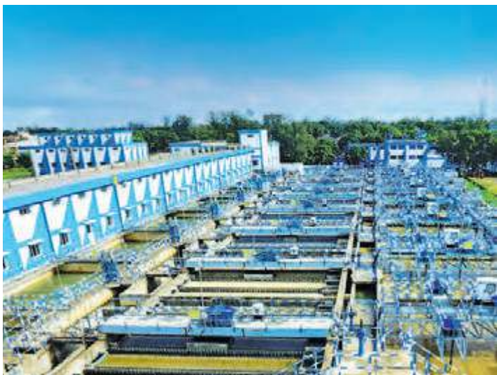
227 MLD Water Treatment Plant, Kolkata, West Bengal
