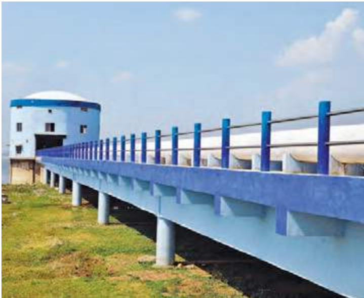
Medak and Sangareddy Water Supply Project
