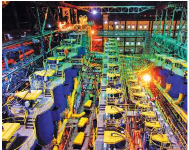
Lead-Zinc Beneficiation Plant, HZL SK Mines, Dariba
