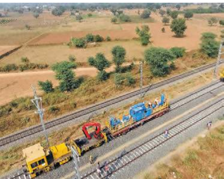
First-in-India: Mechanized simultaneous stringing of conductors at Western Dedicated Freight Corridor
