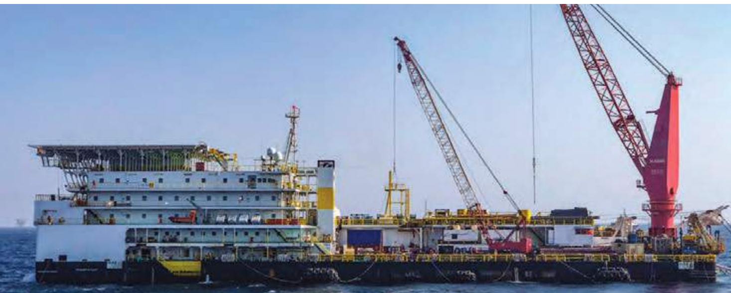
LTB 300, a pipelay-cum-work barge undertaking offshore installation
