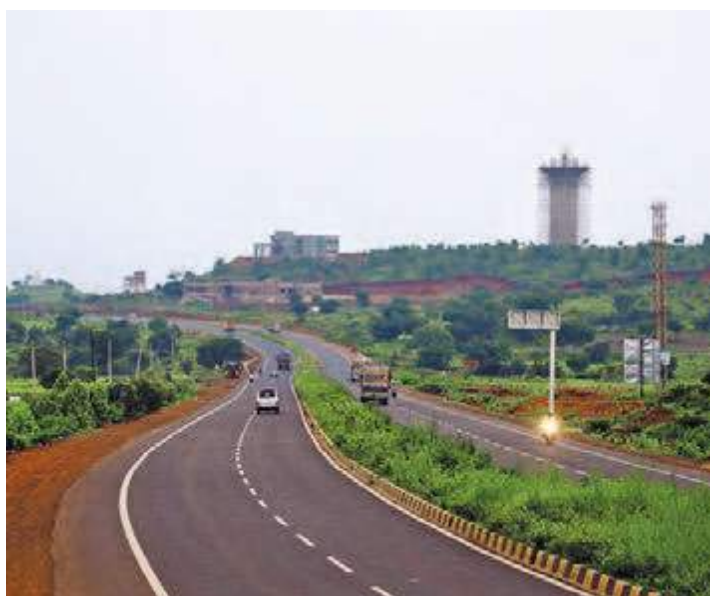
Solapur-Sangareddy Road Project
