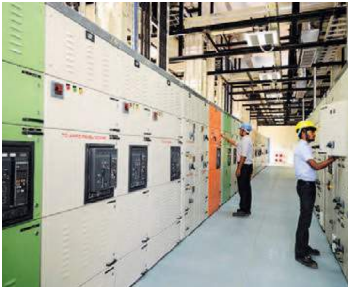
Switchboard installation at a national infrastructure site
