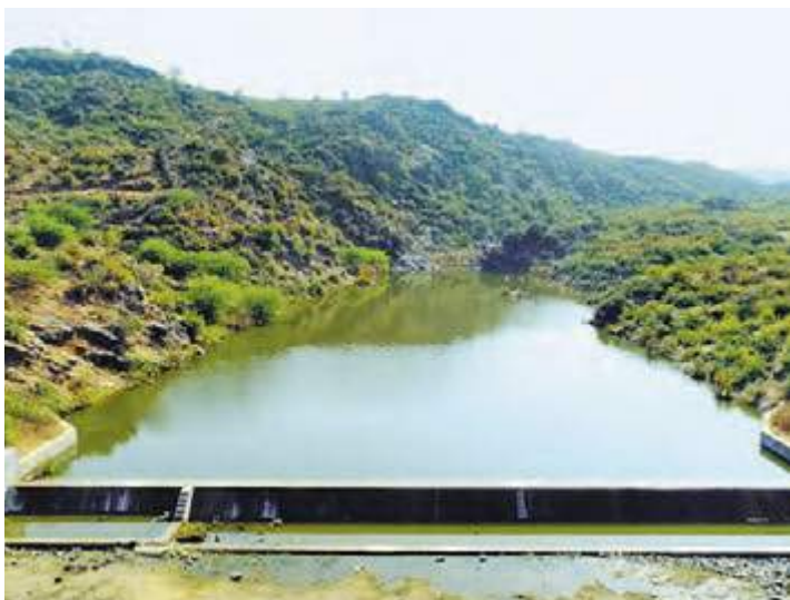
L&T has built over 200 check dams in water stressed areas
