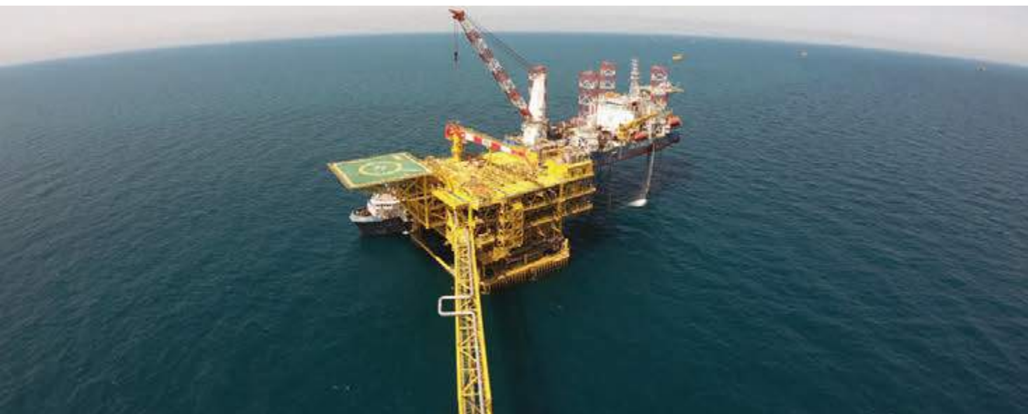
A fully-integrated gas platform - the heaviest in Saudi Aramco's history - installed by float-over method at Hasbah Field in Saudi Arabia
