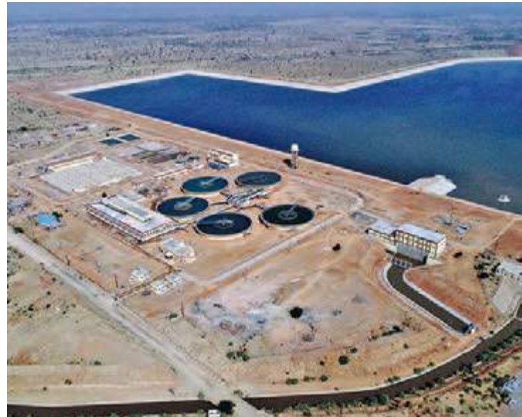
Overview of Nagaur 250 MLD Water Treatment Plant and 5310 ML Raw Water Reservoir
