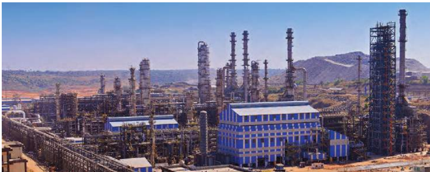
Mangalore Aromatic Complex for ONGC-Mangalore Petrochemicals Limited, India
