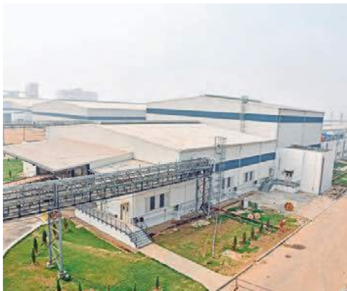
ITC Food Manufacturing and Logistics Facility, Kapurthala
