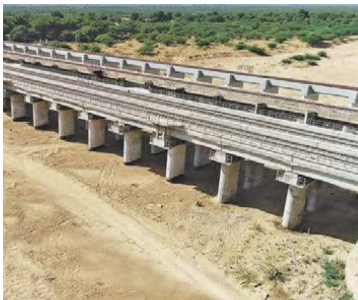
A rail bridge on the Western Dedicated Freight Corridor section being built by L&T
