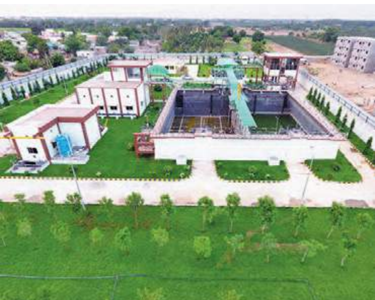
5 MLD Sewage Treatment Plant, Nellore
