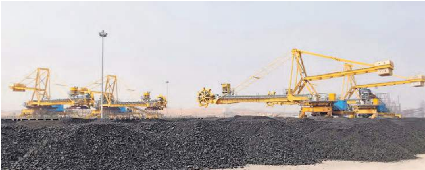
Stacker Reclaimers at work at Suratgarh Power Plant
