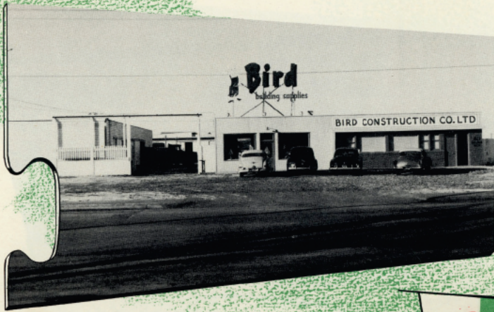
The Lethbridge branch is the centre of the company's extensive operations in southern Alberta. J. O. Langley is branch manager. The present premises were built in 1951 when the firm outgrew its former plant here.
