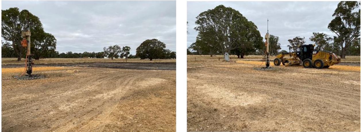
Figure 8: Killanoola site works, January 2023
