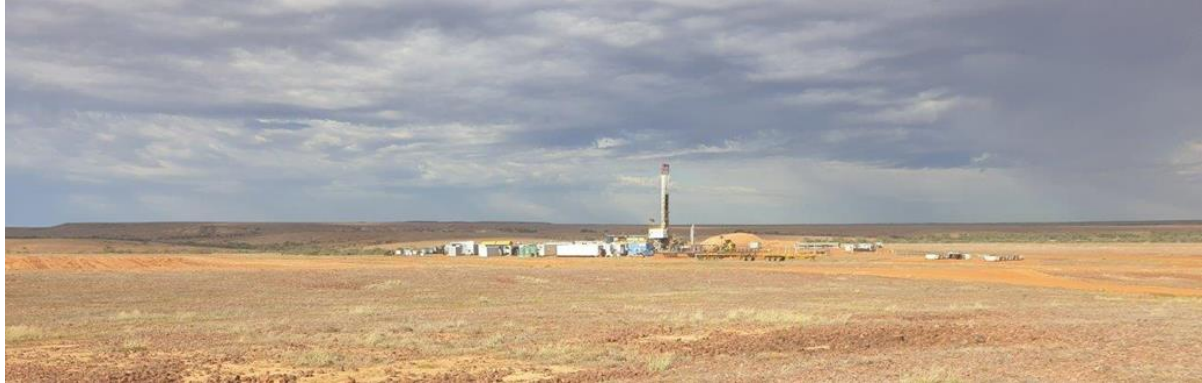
Figure 2: Yarrow 3 Well activity site (Credit:Santos)
