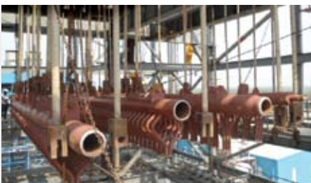
Chennai II Boiler under construction
