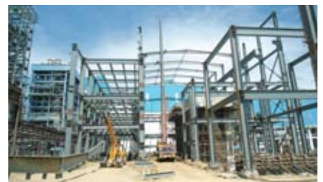
Chennai II Power House under construction
