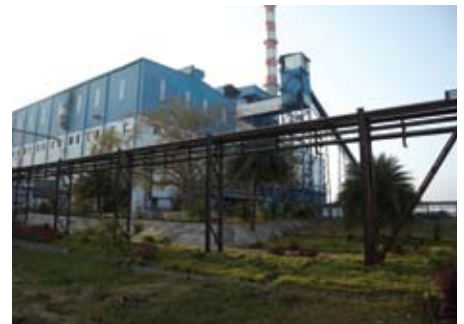
Coal conveyor belt for Chennai I
