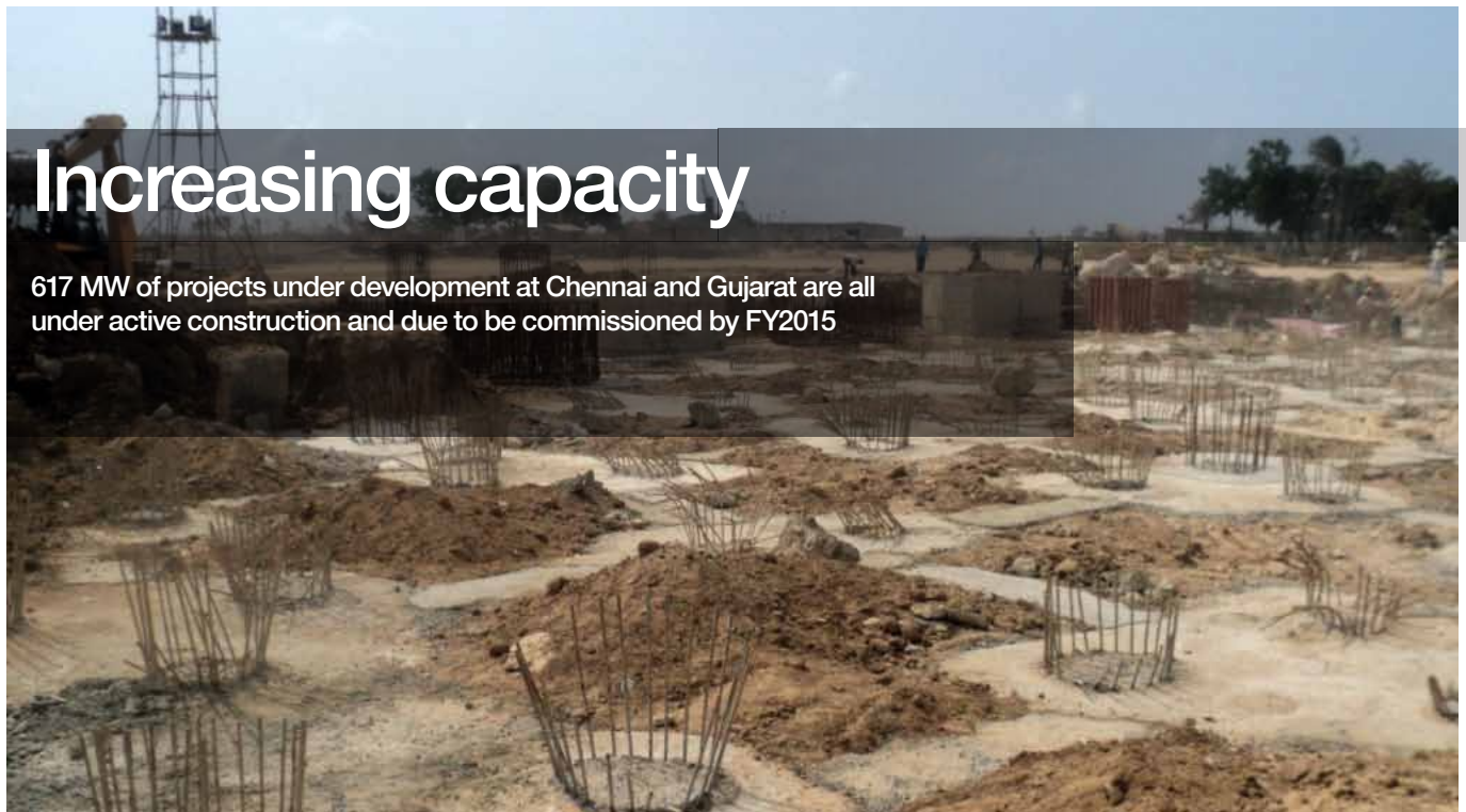
Gujarat boiler foundation work in progress
