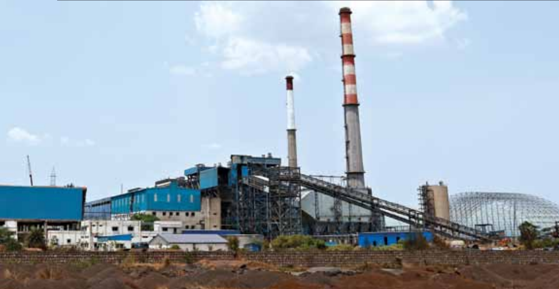
View of the Chennai site showing Chennai I and ongoing construction
