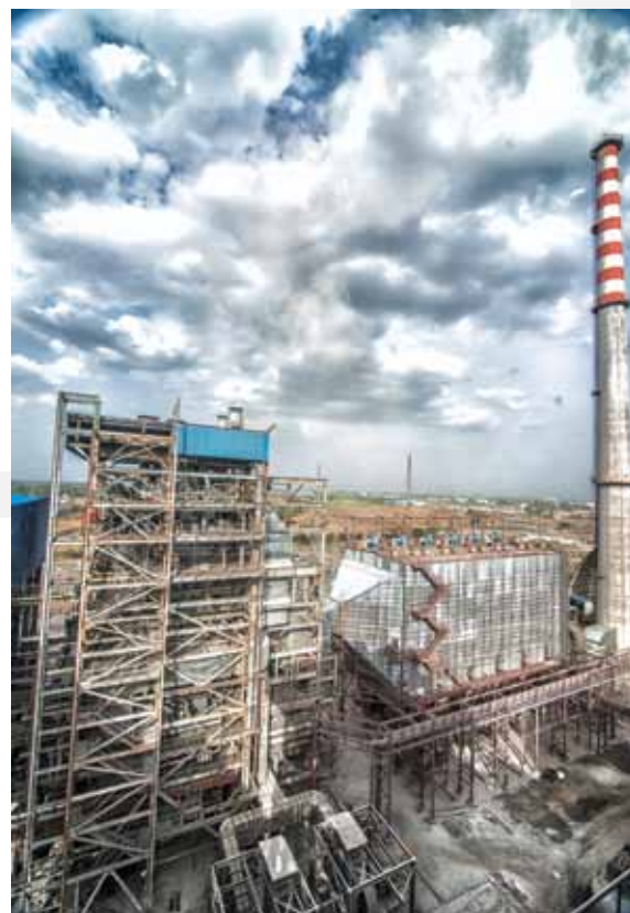
Chennai III near completion
