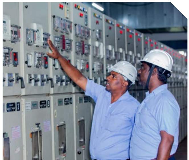
▲ Inspection work on relay panel
