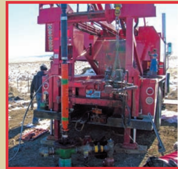
Flotek Pump Services' tools being inserted into a gas well.
