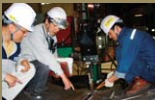
Instruction of improved auto-welding machine operation.
