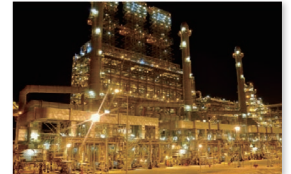
View of the completed Coker Unit
