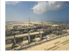
2004 Order awarded for Qatar-gas II LNG Project in Qatar, the largest LNG plant in the world
