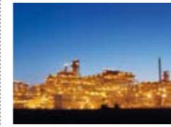
2003 Order awarded for Sakhalin II LNG Project by Sakhalin Energy in Russia, the first LNG plant in Russia
