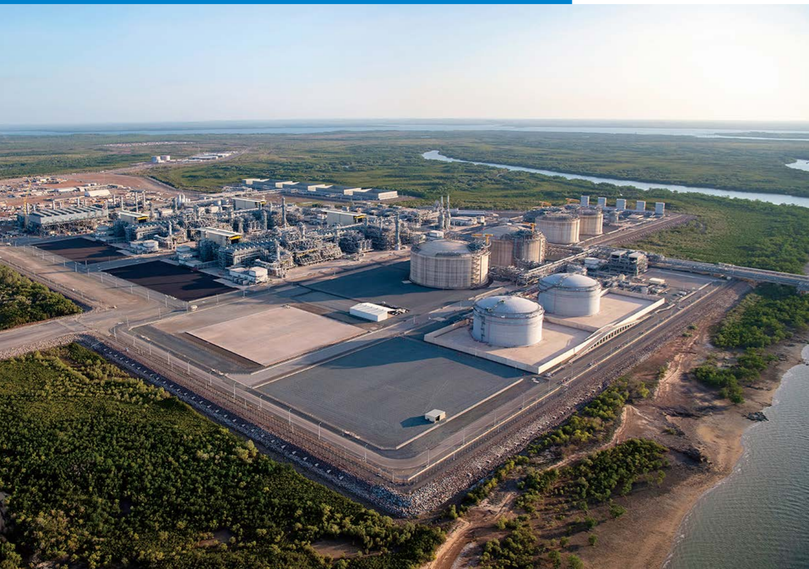
Photo courtesy of INPEX: Ichthys LNG Onshore Processing Facilities at Bladin Point near Darwin, Australia
