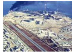
1976 Completion of LNG plant for Abu Dhabi Gas Liquefaction in UAE
