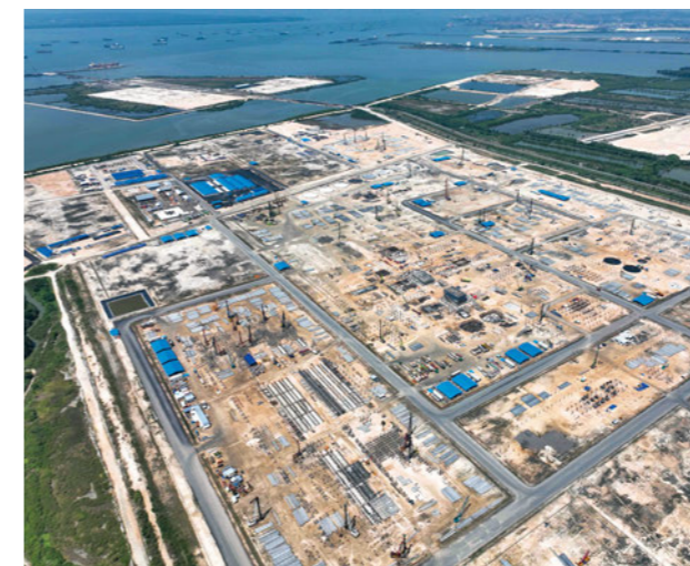
Overview of the plant under construction Courtesy of P.T. Freeport Indonesia
