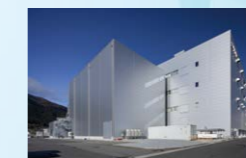
A vaccine constituent manufacturing facility constructed by Chiyoda for Shionogi
