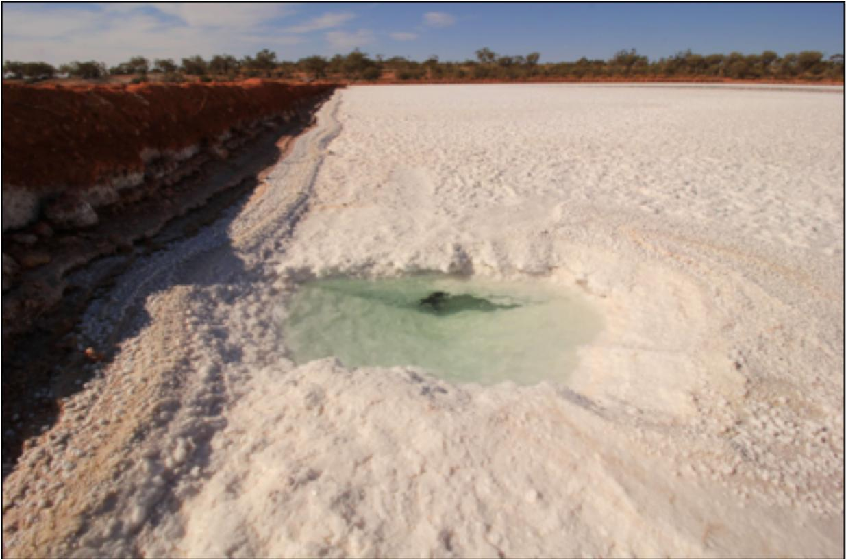
Figure 3: On-playa trial pre-concentration pond demonstrated low-cost, efficient lateral seepage barrier construction techniques, using the highly stable and easily accessible playa perimeter
